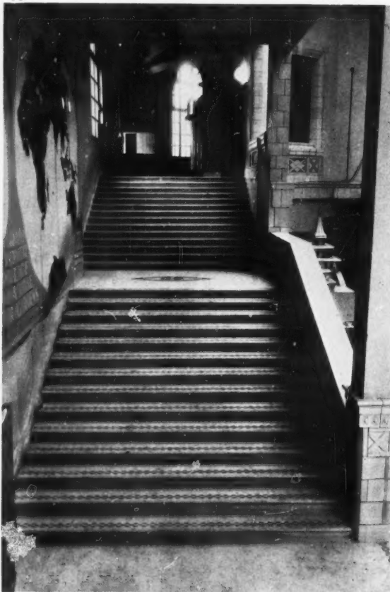
The Marble Terrazzo Grand Staircase at the New Olympia Winter Gardens, Blackpool.
