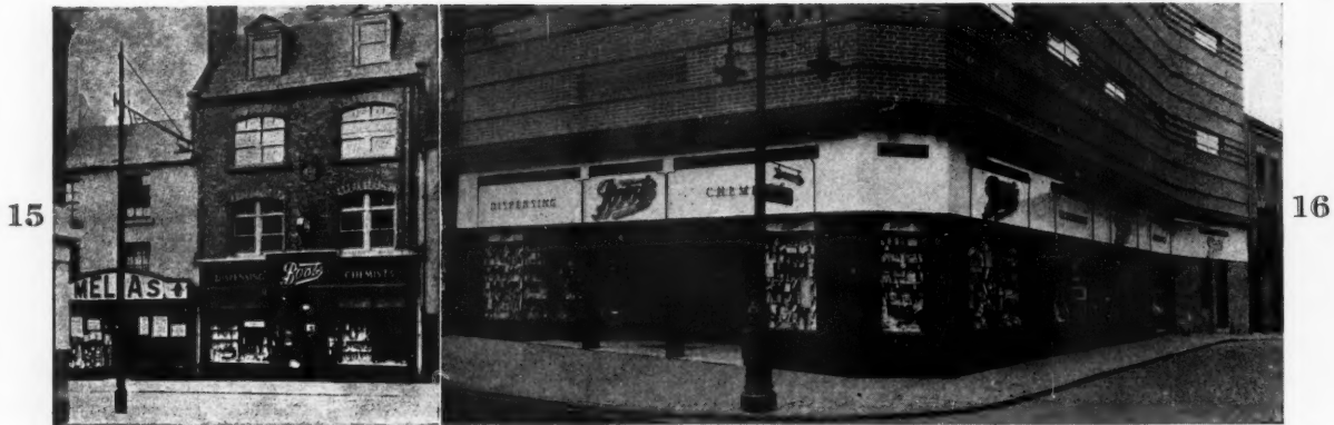
15, 16, 17. Shop Fronts for Messrs. Boots. Designed by Percy Bartlett. In 15 can be seen their early standard fascia, and in 16 and
