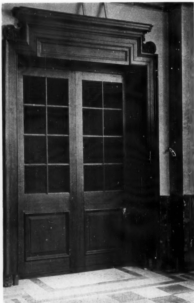
Photograph taken during erection of a pair of doors in Austrian Oak at the N.P. Bank, Thames House.
