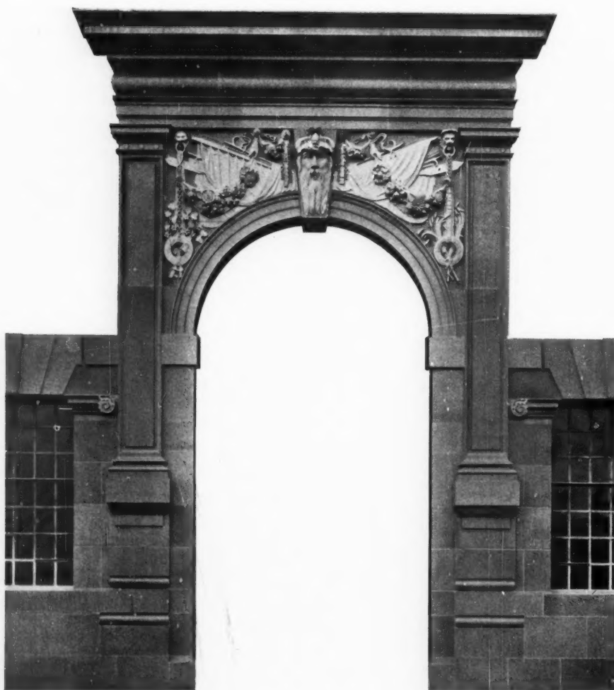
One of the eight principal entrances to Thames House showing typical polished and carved granite work.
