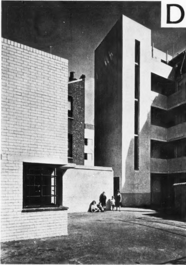
New flats in Silchester Road, North Kensington, W. Messrs. T. Smith Shearer and S. Cameron Kirby, A.A.R.I.B.A. (Architects).
