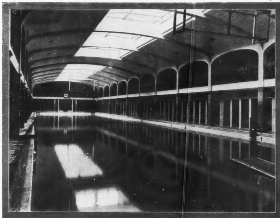
THE RECONSTRUCTED WHITE ROCK SWIMMING BATH, HASTINGS SIDNEY LITTLE, Assoc.M.Inst.C.E., BOROUGH ENGINEER.
