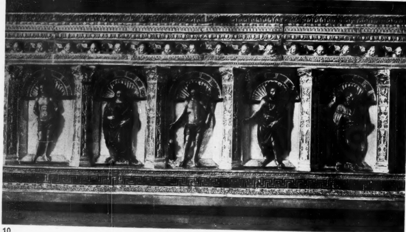
(8) The terra-cotta architrave of a doorway near Milan. This architrave is built in three courses—the inner band bearing the leaf ornament, the ornately modelled central detail and the egg and dart crown, each consisting of a separate series of blocks. (9) CREMA. Detail of terra-cotta ornament of the cathedral, dating from the thirteenth century. (10) FLORENCE. Altar piece of glazed polychrome terra-cotta by Giovanni della Robbia, dating from about 1500, now in the National Museum.
