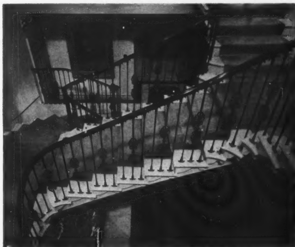
The MAIN STAIRCASE looking down to the ground floor from the first-floor gallery. The balusters are of yellow bronze and the rail of red mahogany. The walls and dome are painted cream.
