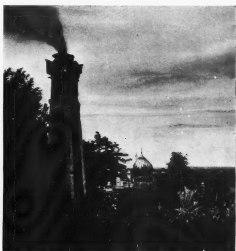
THE WELLINGTON PILLAR on the bank in which is embedded the south-west front of the house. This monument is of Cotswold stone to which is affixed lead plates bearing the names and dates of all Wellington's battles. The pillar also acts as a chimney for the heating apparatus of the orangery beyond and below it; a useful suggestion for War Memorial Committees.
