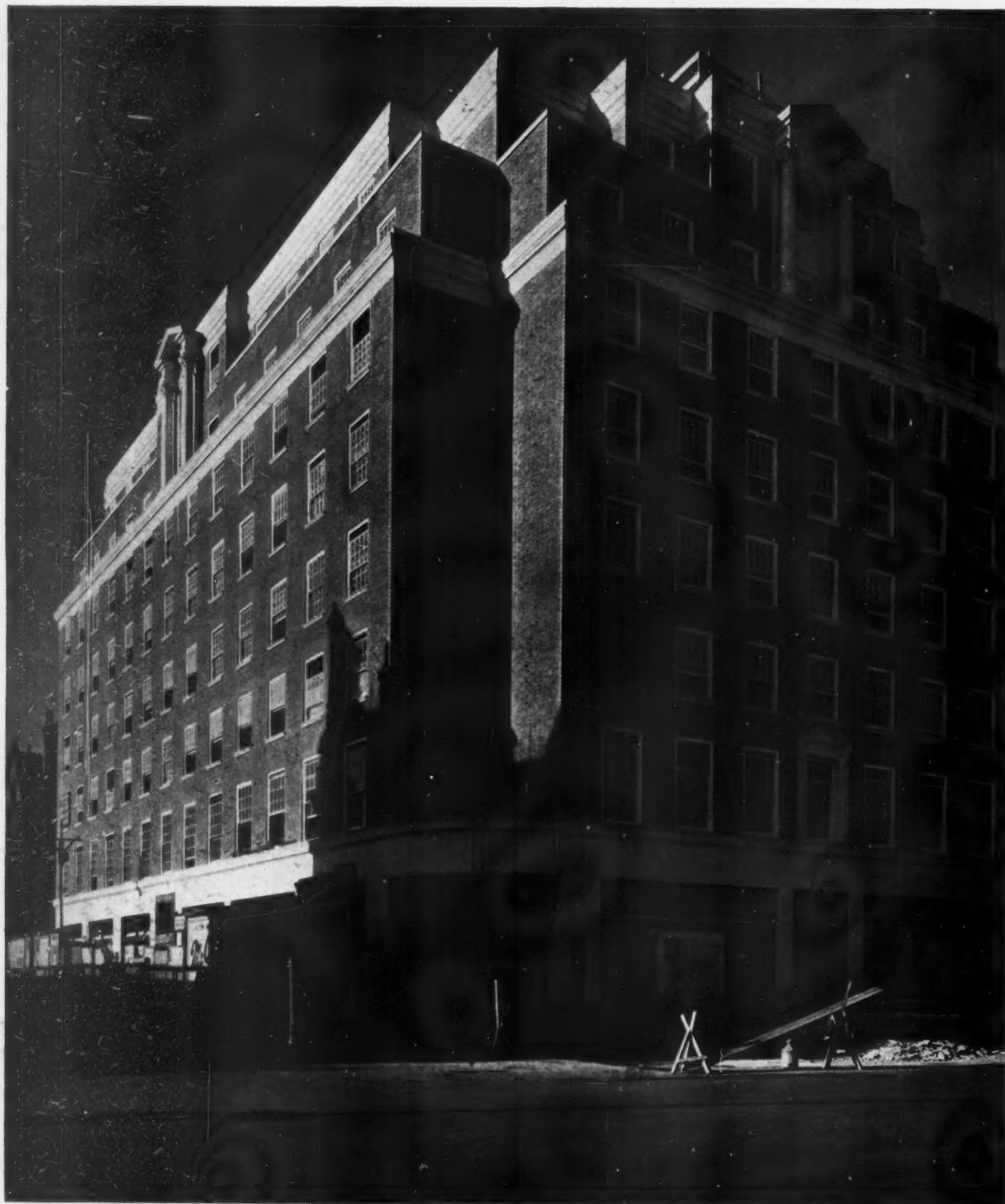
GAMAGE'S West End Store, in Hereford Gardens, Messrs. Joseph, in association with Sir Edwin Lutyens, Architects, is executed in 2-in. red bricks with stone dressings to harmonize with the other new buildings on the Grosvenor Estate. The north-east corner of the building, where Park Street meets Oxford Street (1), shows fine masses of brickwork and the unpierced surfaces rising in Lutyens's blocks to the sky.
