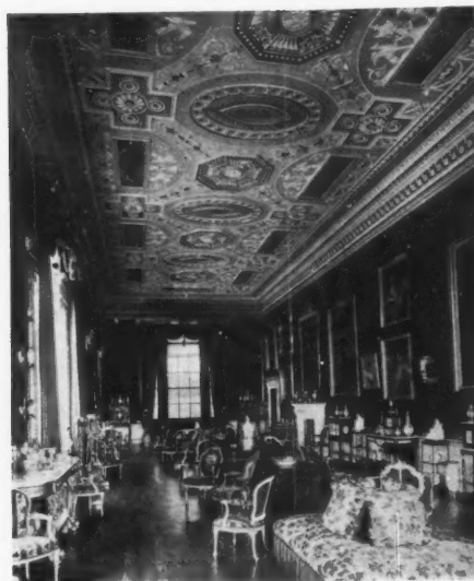
c. 1770. King: George III. 1772. FIG. 590.—Harewood House, near Leeds. Robert Adam, Architect.
