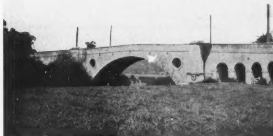
New Bridge, near Corston.
