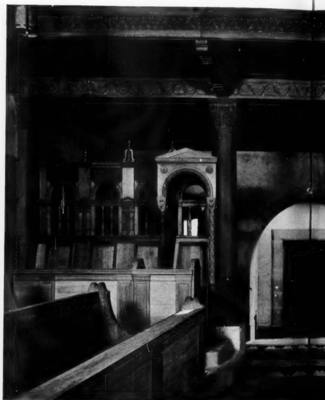
The west end of the Chapel, showing Screen, carried out in Selected
