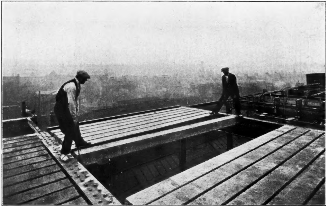
VIEW SHOWING 17 FT. LONG HOLLOW SIEGWART BEAMS BEING LAID.
