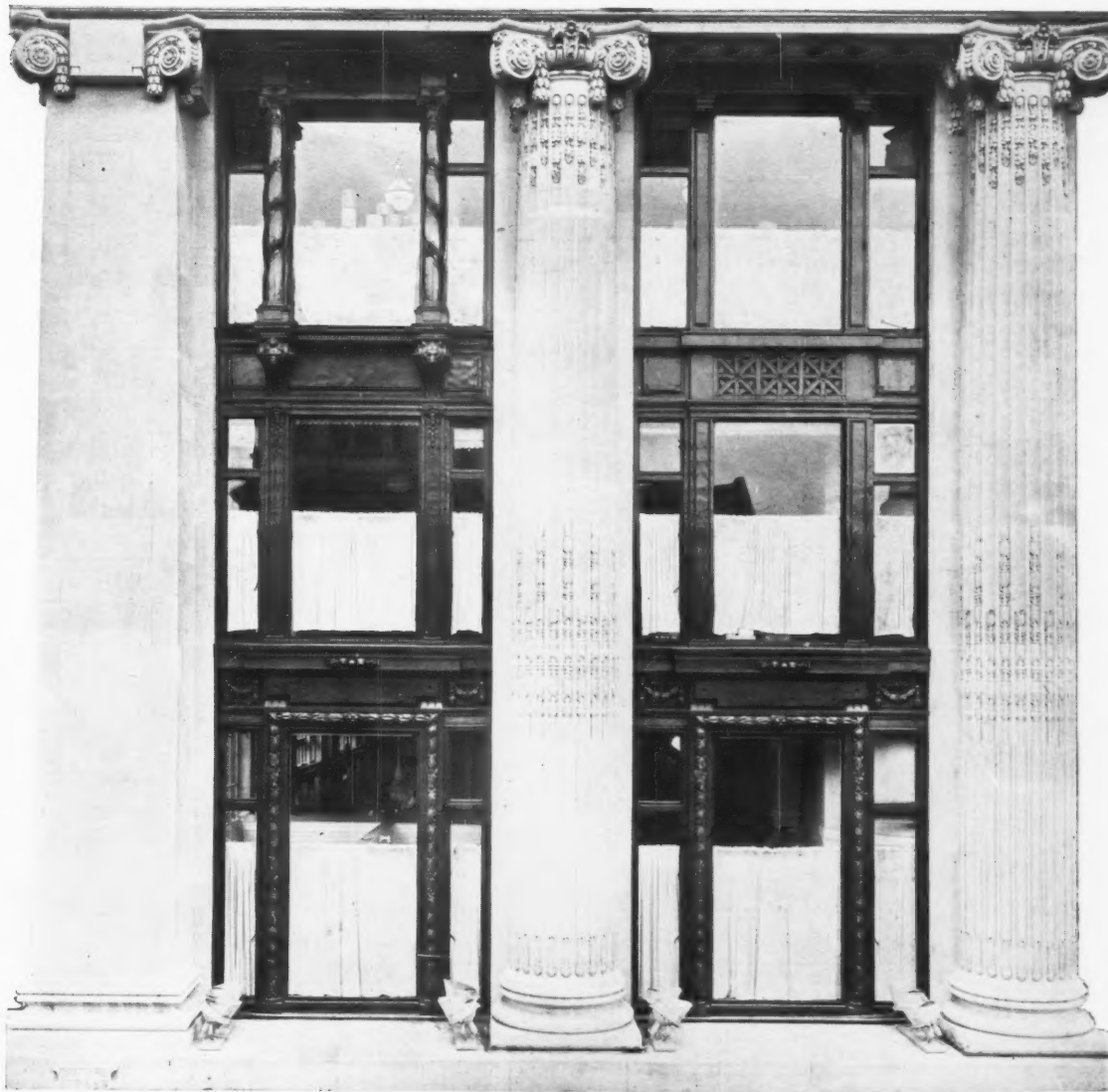
DETAIL VIEW, MESSRS. SELFRIDGE'S BUILDING, LONDON.
