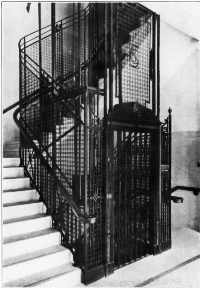
LIFT ENCLOSURE, NEW CO-OPERATIVE STORES, SCUNTHORPE. Architect: W. A. Johnson, Esq., C.W.S. Architects' Dept.
