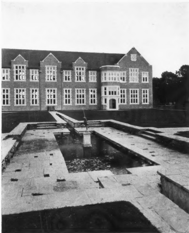
NEW SCIENCE BLOCK, CHRIST'S HOSPITAL, HORSHAM. SYDNEY TATCHELL, F.R.I.B.A., ARCHITECT.
