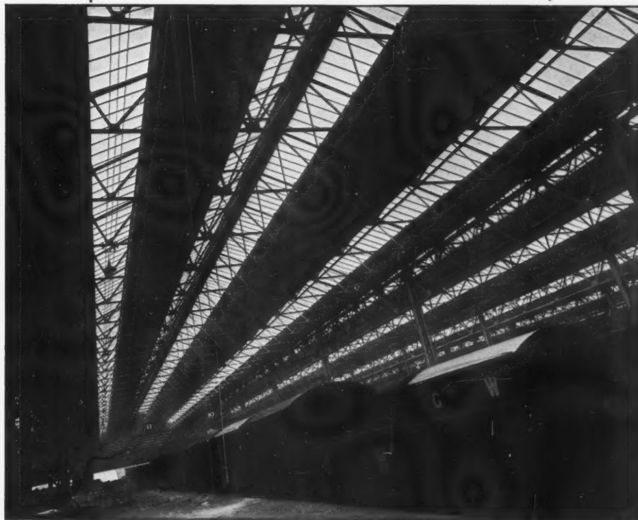
"Eclipse" Patent Roof Glazing at the G.W.R. Goods Sheds, Paddington.
