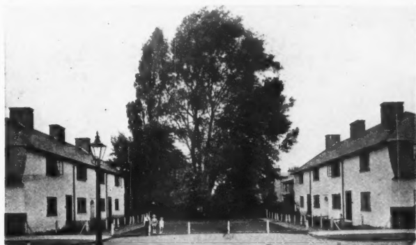
Here is some good L.C.C. housing at Roehampton
