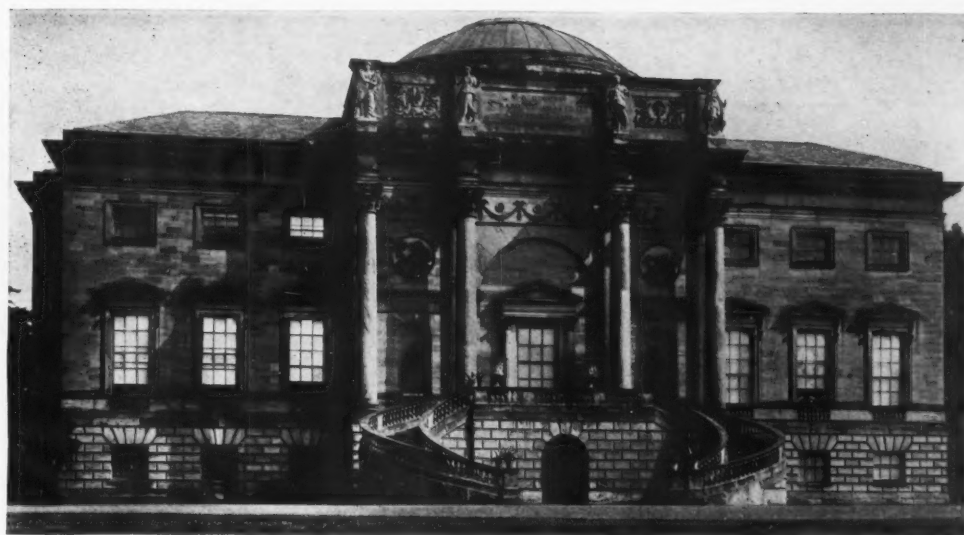
FIG. 524.—The south front of the centre block of Kedleston. Robert Adam, Architect.
