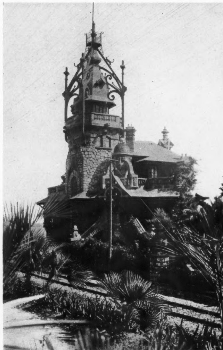
A House between Juan-les-Pins and Cannes, largely executed in glazed tiles and glazed bricks.
