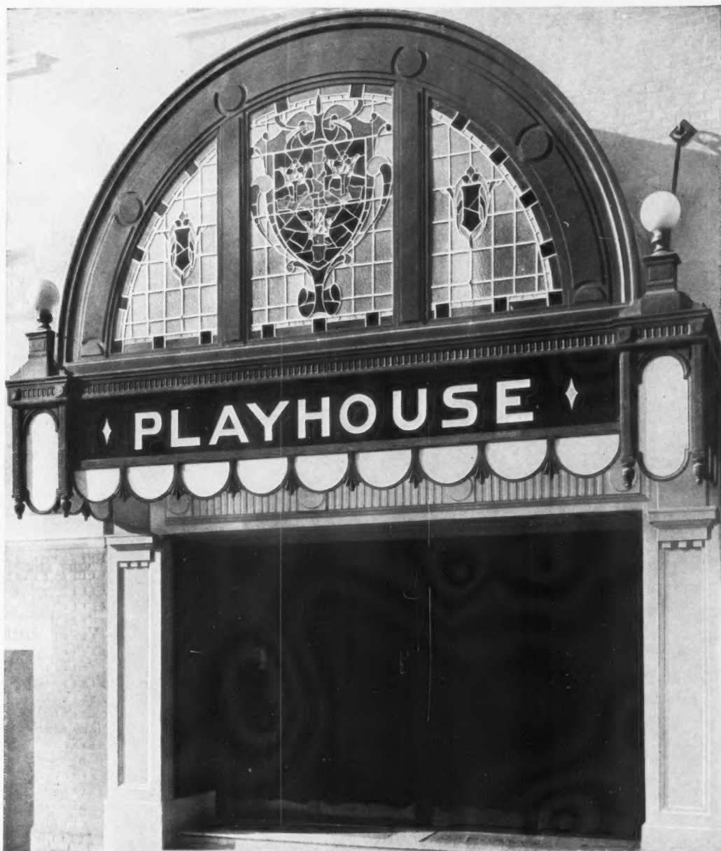
CAST IRON CANOPY, THE PLAYHOUSE, COLCHESTER.
