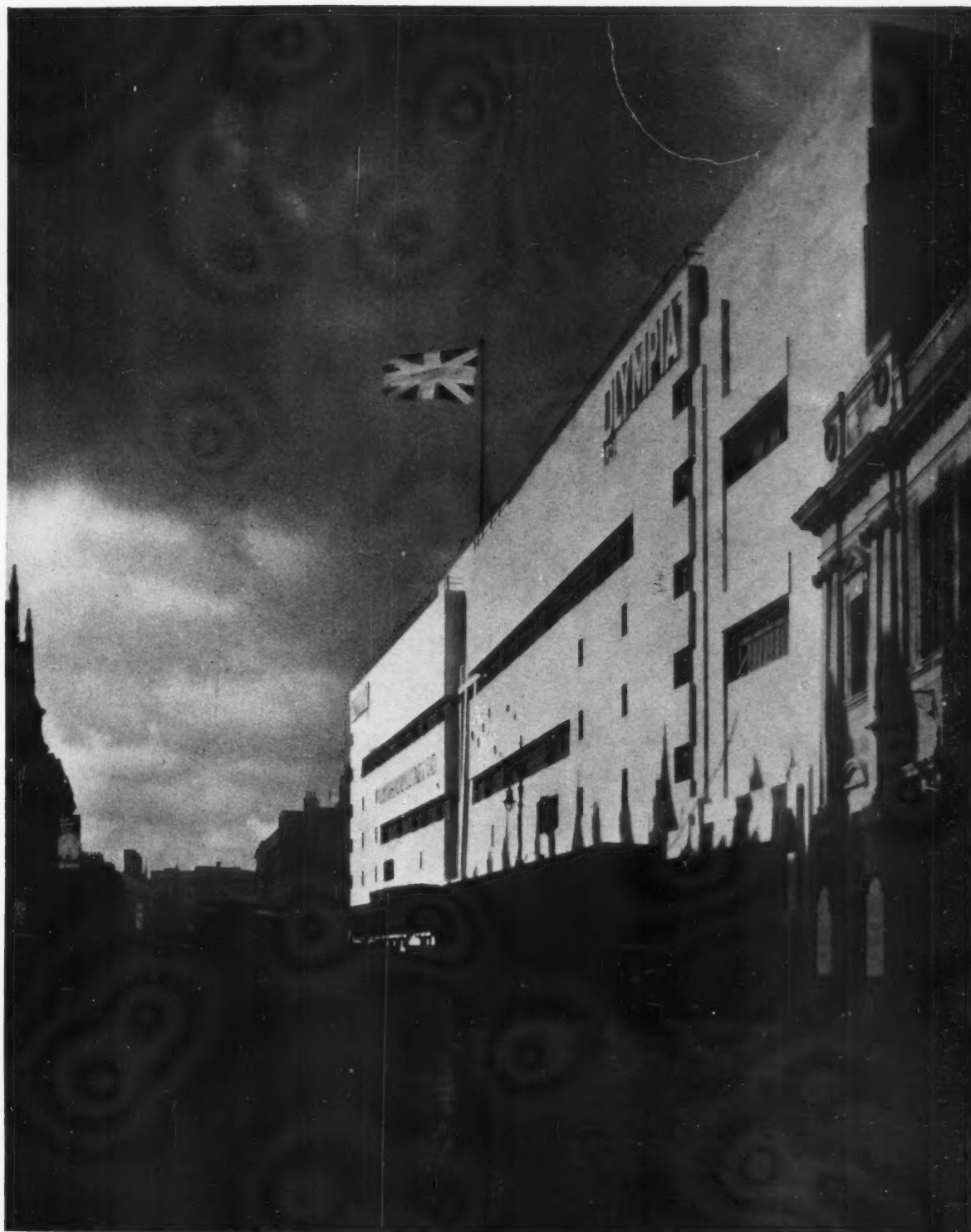
✓ Empire Hall, the new extension to Olympia, London, from Hammersmith Road. Joseph Emberton, Architect. This is the first multi-storied exhibition building to be erected in England. The horizontal treatment of the façade provides permanent fixings for the advertisement of exhibitions.
