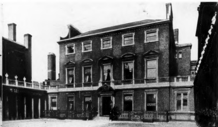
FIG. 461.—Chesterfield House. Isaac Ware, Architect. King: George II.
