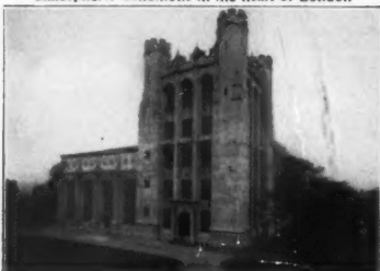
BRISTOL UNIVERSITY Keystona chosen for ceilings and walls. Keystona concrete Paint used on surfaces finished with Portland Cement
