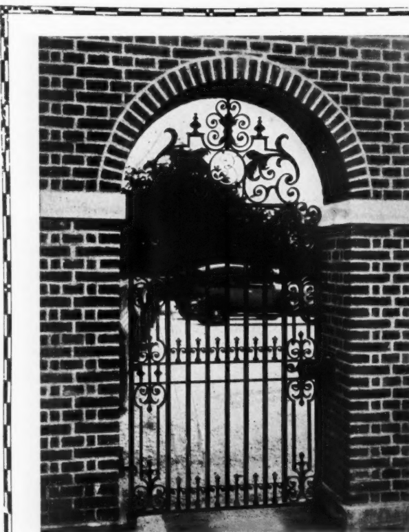
ARCHITECT: E. VINCENT HARRIS, ESQ., F.R.I.B.A.
