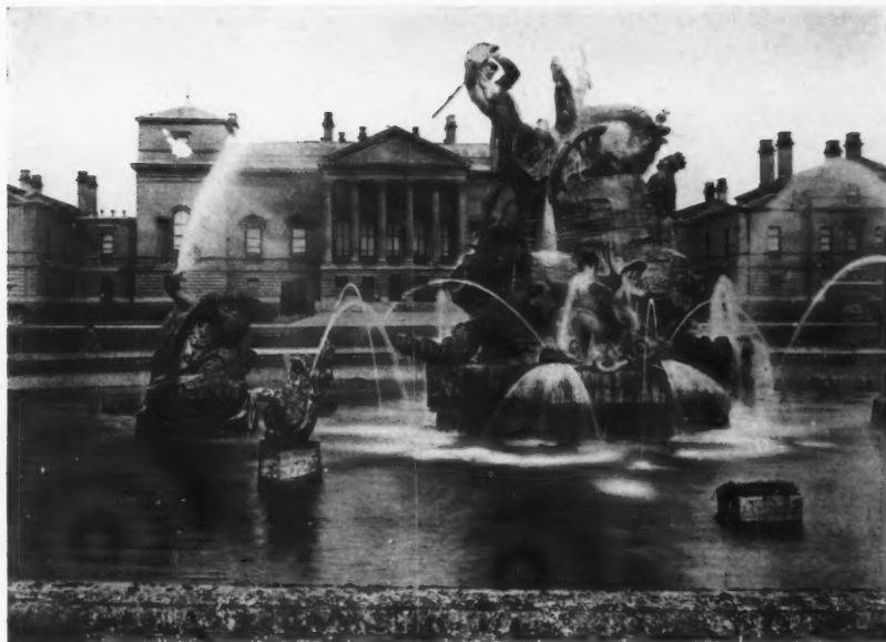
c. 1734-51. King: George II. FIG. 456.— Perseus and Andromeda . Fountains on the terrace on the south front, Holkham Hall, Norfolk. William Kent, Architect.
