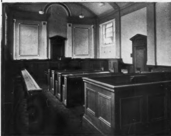
Court Fittings, Gray's New Police Courts.
