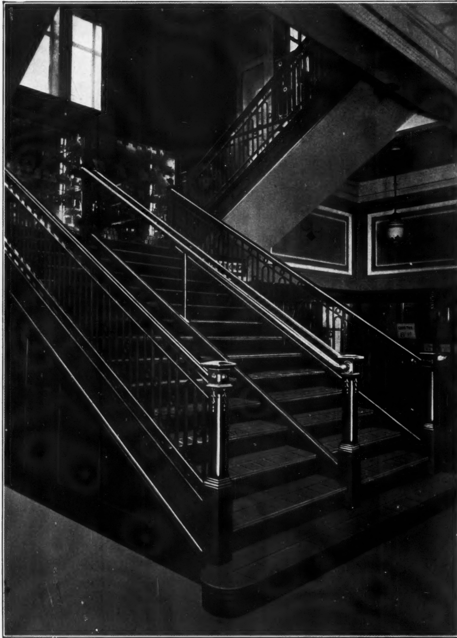
Haywards Type No. 161 Internal Staircase erected for Messrs. Woolworth Ltd. in London (four Branches), Sunderland, Bradford and Accrington.
