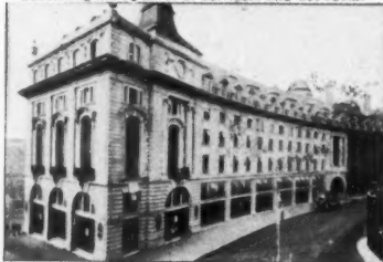
SWAN & EDGAR, LTD., LONDON To keep down the heavy cost of redecorating, a paint that was easily washable and would not shell was needed. That is why Keystona was used
