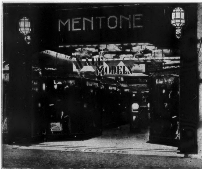
A Modern Shop-front in Oxford Street executed in Black Alabaster Glass by Fredk. Sage & Co. Ltd. Taperell and Haase, 5 Stratford Place, W.1, Architects.
