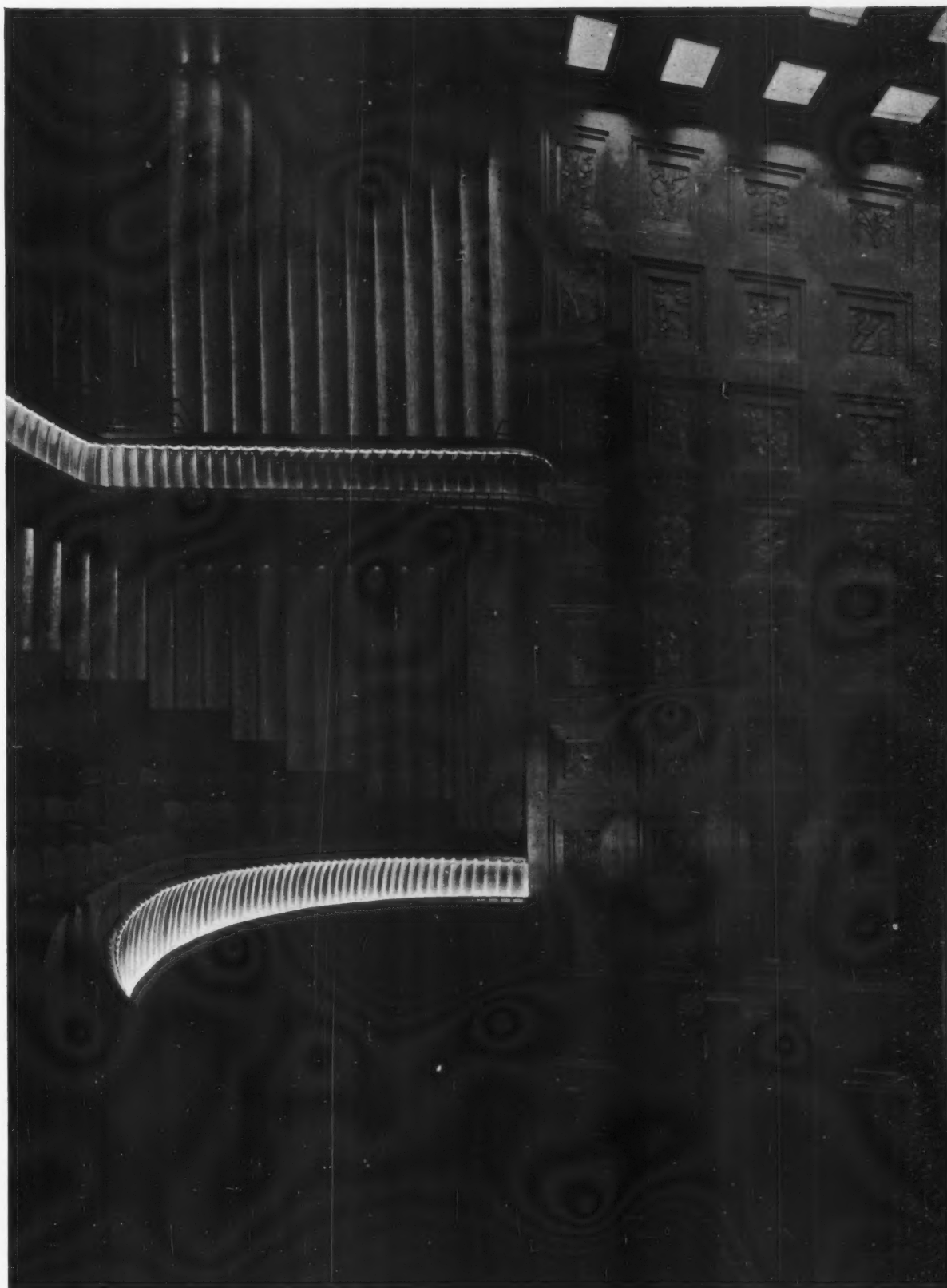
From the ROYAL BOX , showing the junction of the balconies and proscenium coffer framing. The division of the theatre at this point is deliberate so that the framing is related to the stage and brings the audience nearer. The whole is in gold, but round the top of the balconies is a strip of coral velvet.
