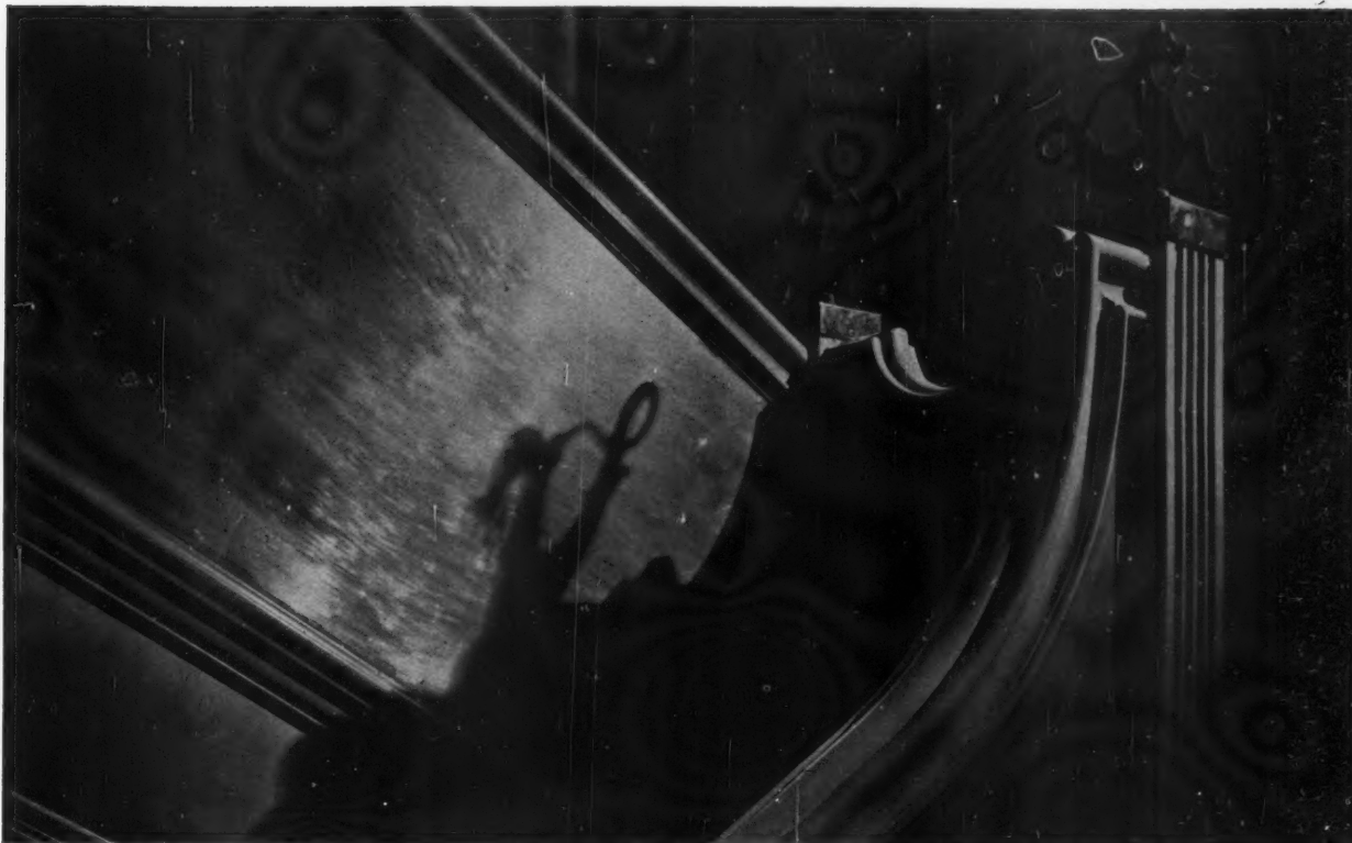
The polished copper stair balustrade and the newel-caps on the half-landing of THE STAIRCASE . The dado, newels, string and handrail are lavender cellulose. The sea-horses on the newel-caps are brass on black nickelled bases. The stair-treads and risers are laid with maroon rubber with a border of Naples yellow.
