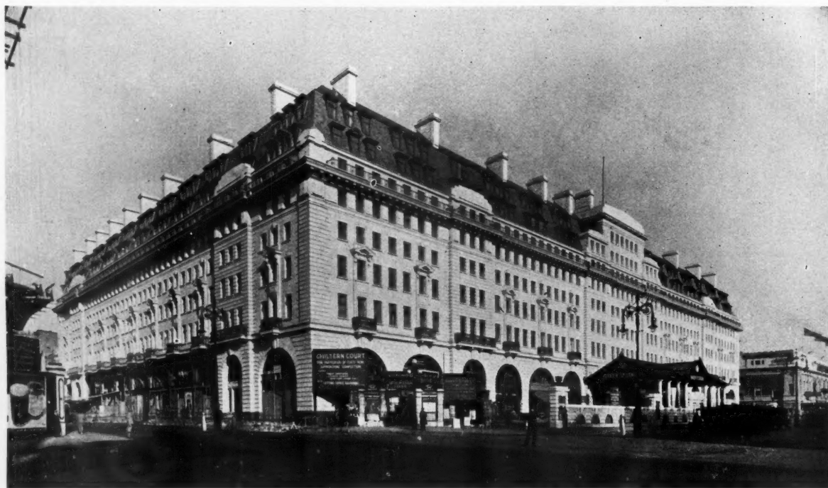
CHILTERN COURT FLATS.
