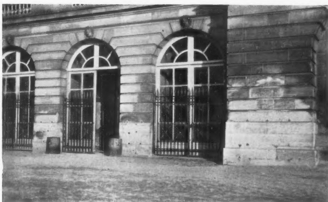
Building treated with KNAPEN SIPHONS. Notice the wall dried out where siphons are inserted.
