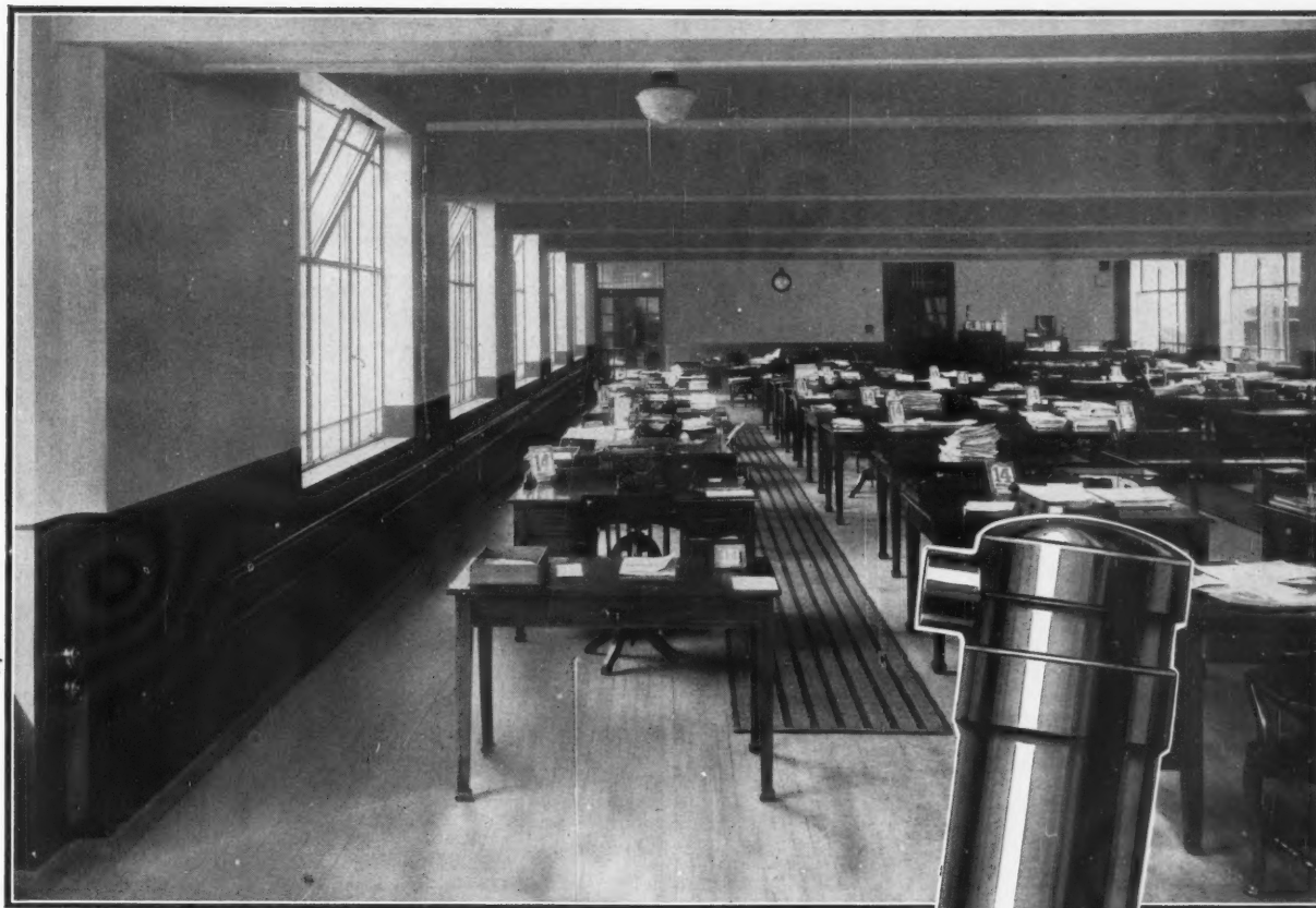
'Unity' Electric Heaters with Thermostatic control * in large general office.
