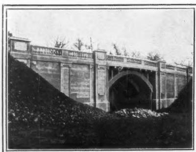
Coombe Dingle Bridge, Bristol
