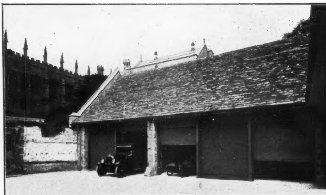
CHRIST CHURCH COLLEGE, OXFORD: GARAGES. Fitted with 12 Kinnear Shutters.
