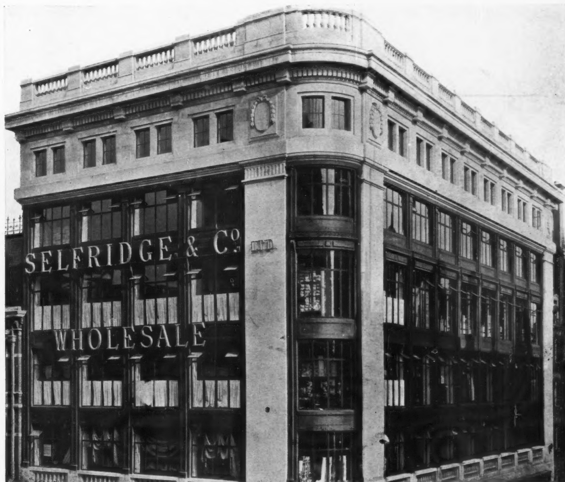
CAST IRON BUILDING FRONT SUPPLIED AND ERECTED AT BUSINESS PREMISES 419 OXFORD STREET, LONDON.
