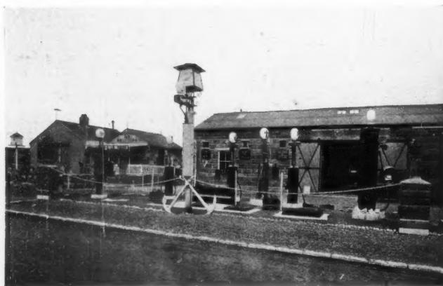
Commonhead, near Swindon, Wiltshire.
