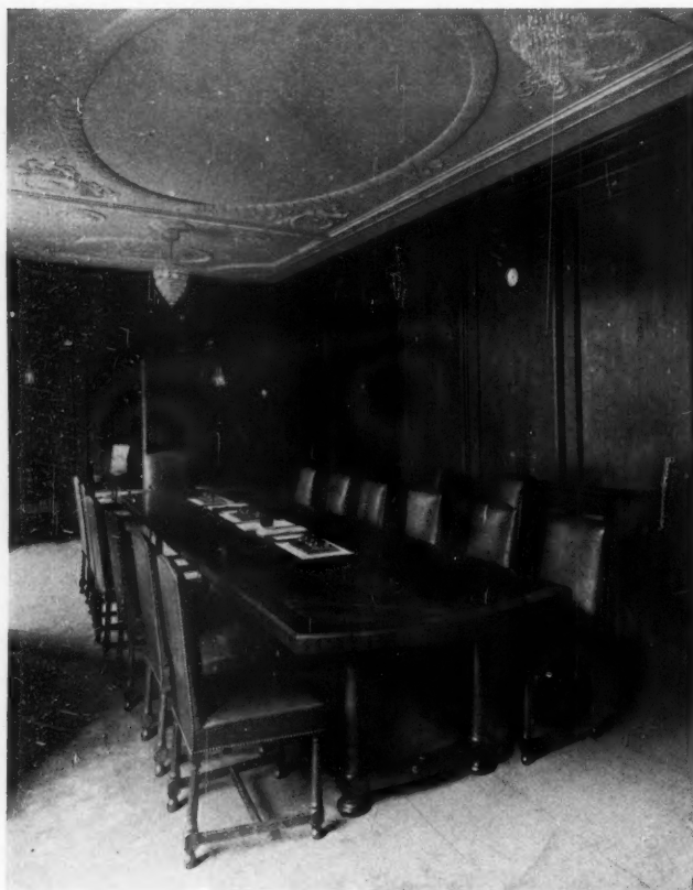
The CONFERENCE ROOM on the second floor. The panelling is in Austrian oak and the plaster ceiling is finely modelled. The furniture is in oak and leather.
