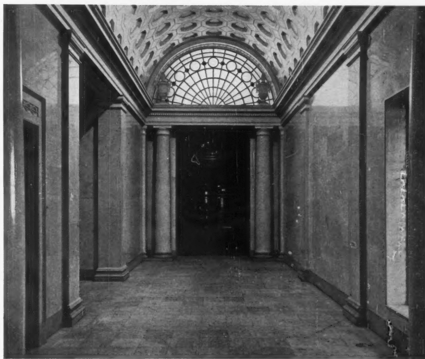
Looking south from the WEST ENTRANCE. The walls and floors are of Subiaco marble and the vault is built of fibrous plaster.
