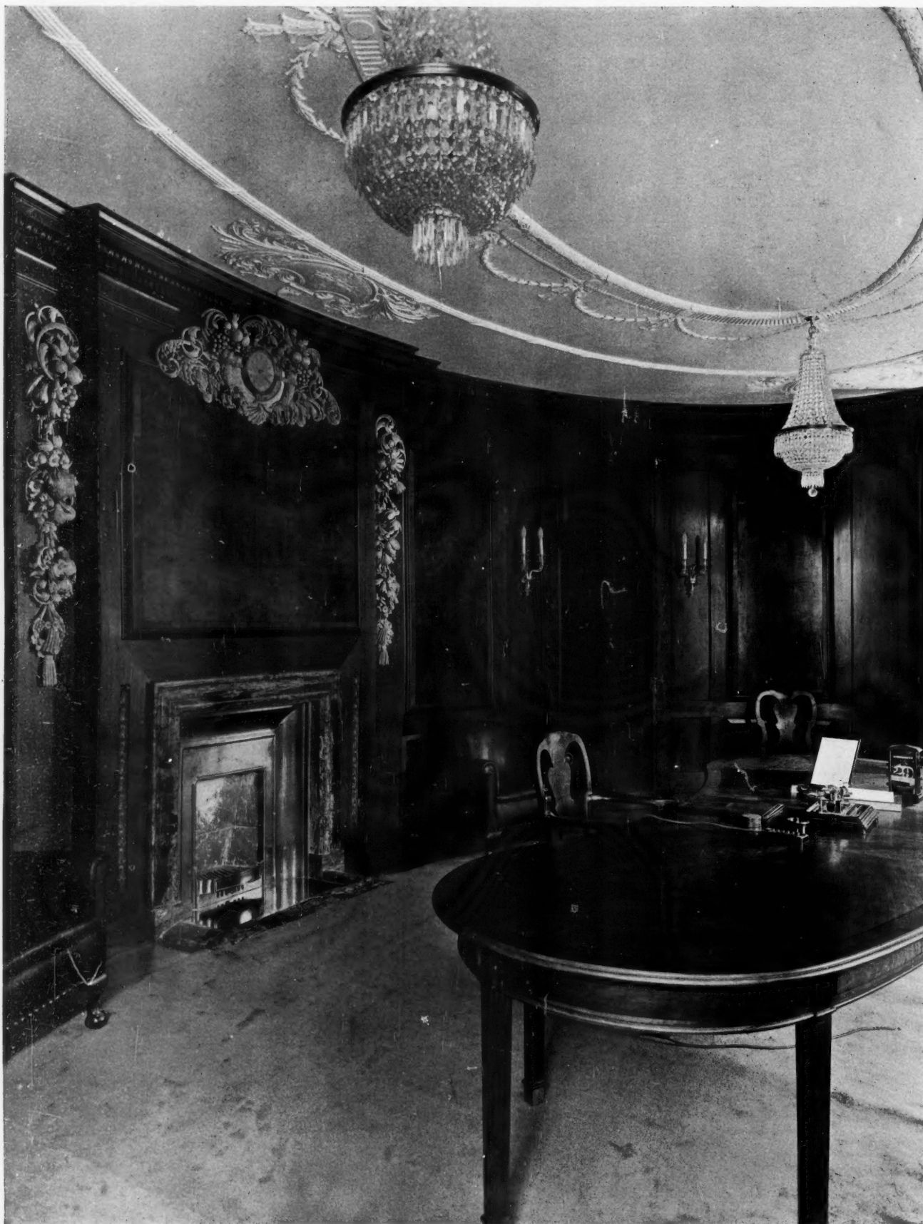
The CHAIRMAN'S ROOM on the second floor. The panelling and furniture are carried out in walnut, and the carving is in limewood. The electric light fittings are of white metal and glass. The fibrous plaster ceiling is modelled in very low relief.
