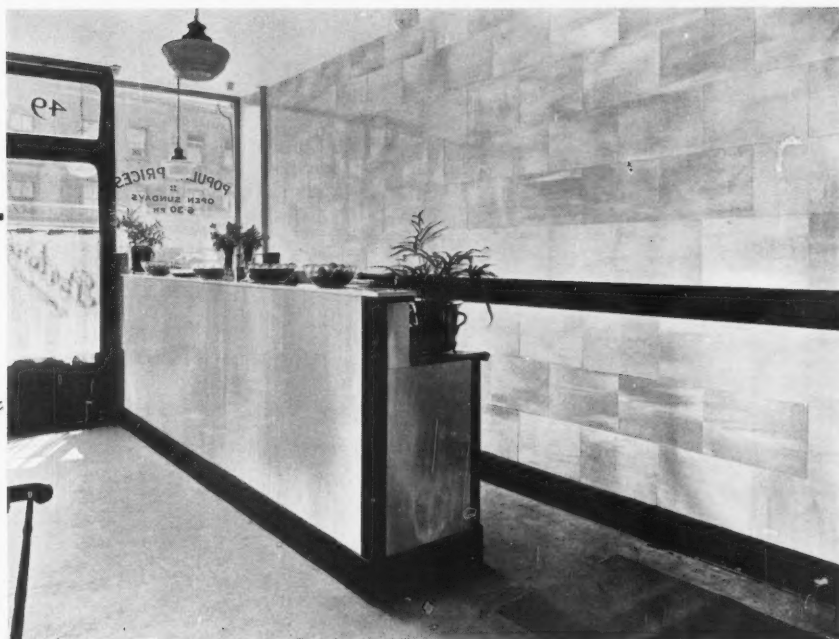
Shop—Walls lined with Pink Marbled Vitrolite pieces, the Counter with panels. Black Vitrolite skirting and dado rails.
