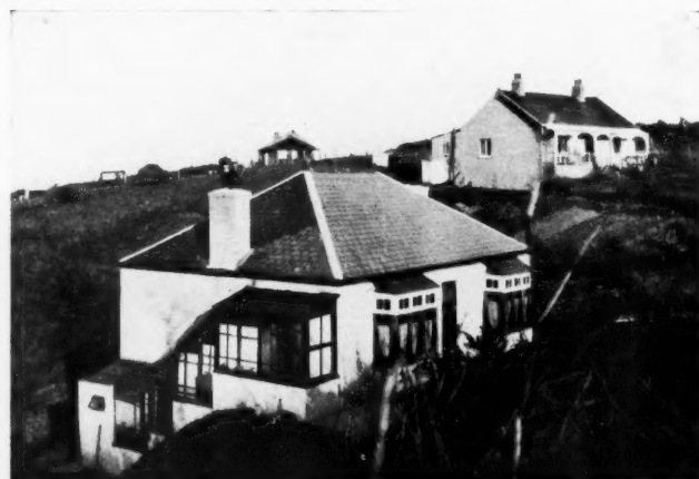
"The right bank of the Yealm slopes precipitously down to the river; and clinging to its face are bungalows, semi-bungalows, and all manner of horrors."
