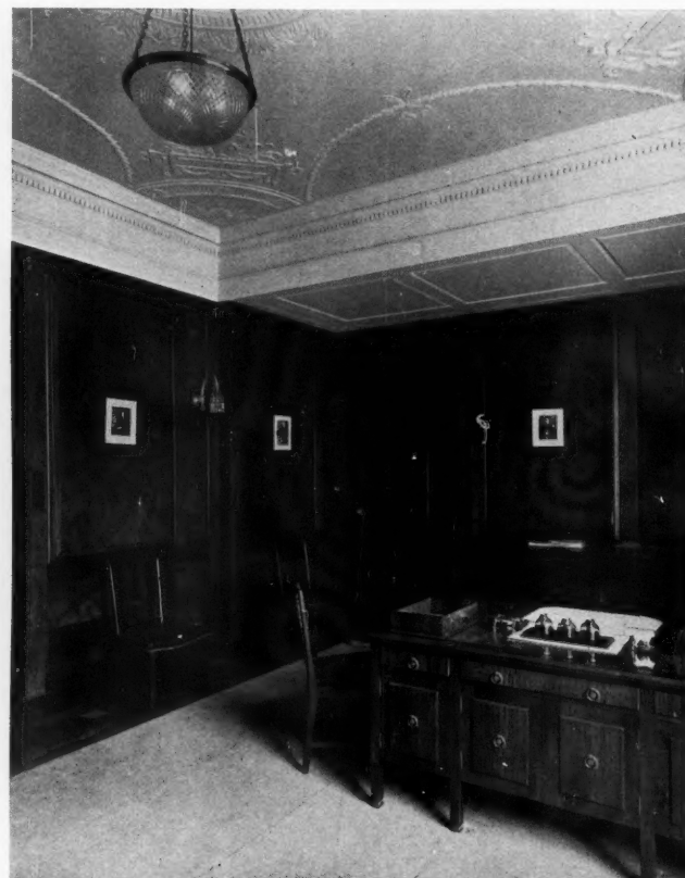
The GENERAL MANAGER'S ROOM on the second floor. The panelling is in sycamore and the ceiling is modelled in plaster. The furniture is of walnut.
