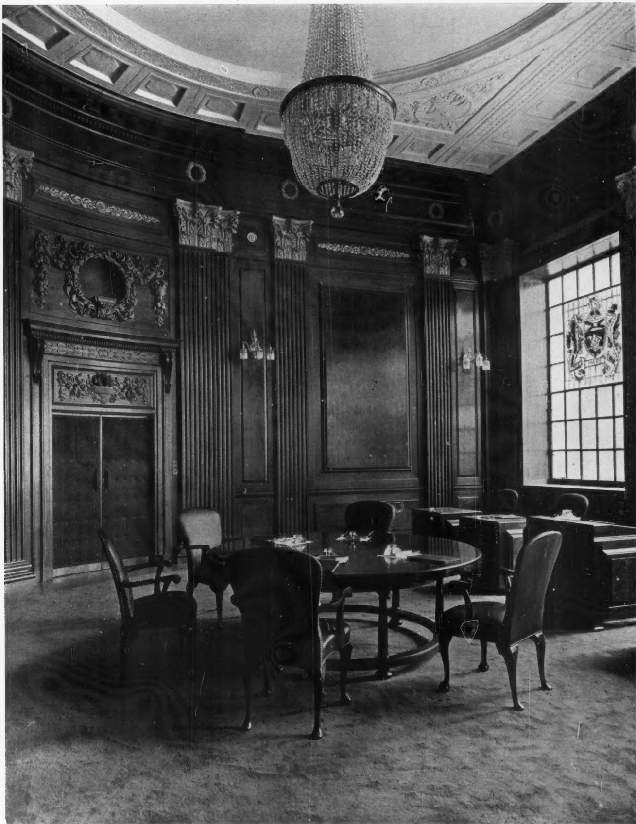
The BOARDROOM on the second floor. The walls are panelled in figured walnut, and the furniture is made of the same wood. The pilaster caps and other carvings are in limewood. The electric light fittings are of white metal and glass. The ceiling is in fibrous plaster.
