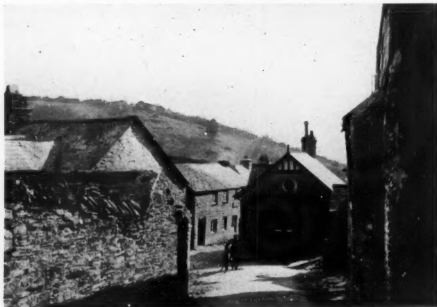
"The cottages are all of limestone, the roofs are slated, and yet the gable of the village meeting place is 'half-timbered'."
