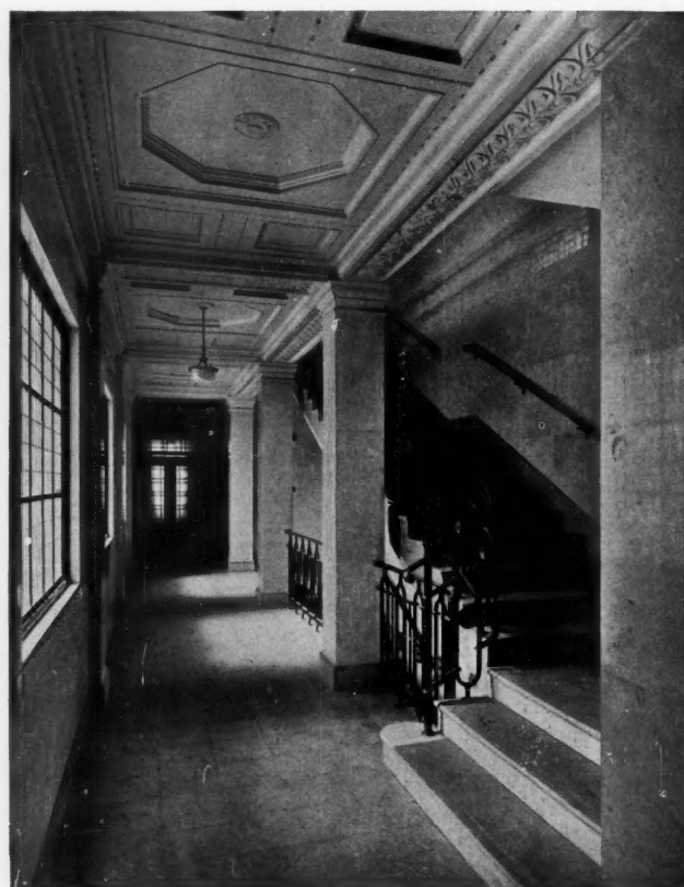
The STAIRCASE on the second floor, looking west. The treads to the stairs are of rubber.
