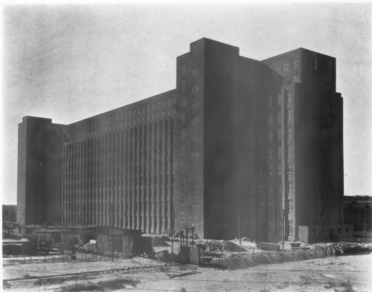
ELECTRICAL WORKS IN BERLIN.
