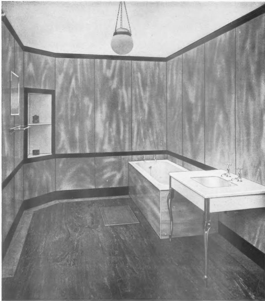
The illustration above shows a Bathroom lined from floor to ceiling with Green Marbled Vitrolite, broken by Black Vitrolite skirting, dado rail and capping. The bath is also enclosed with Green Marbled Vitrolite.
