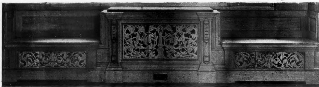
A radiator grille and window seats at 29 Belgrave Square, London. Made from Austrian OAK with CARVED and PIERCED panels and CARVED brackets. Designer : SIR EDWIN LUTYENS, R.A. Craftsman : JAMES WALKER.
