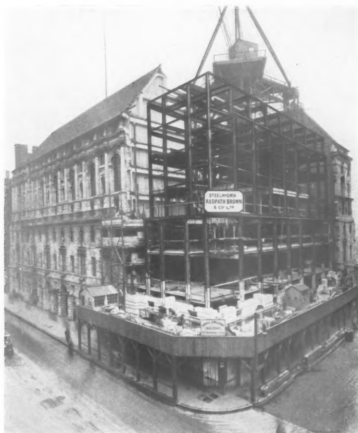
Architect: Sir Edwin L. Lutyens, R.A. Builders: Howell J. Williams, Ltd. Britannic House, E.C. (Erection of Corner Block.)
