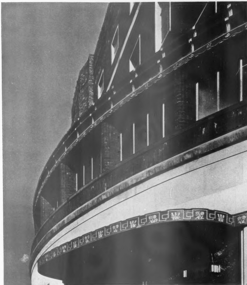
Above : A DETAIL of the segmental BAY in the WEST Front. The decoration is of cast lead, gilded; the small enrichment is composed of a SHELL alternating with a REBUS of the letters R.H.S.
