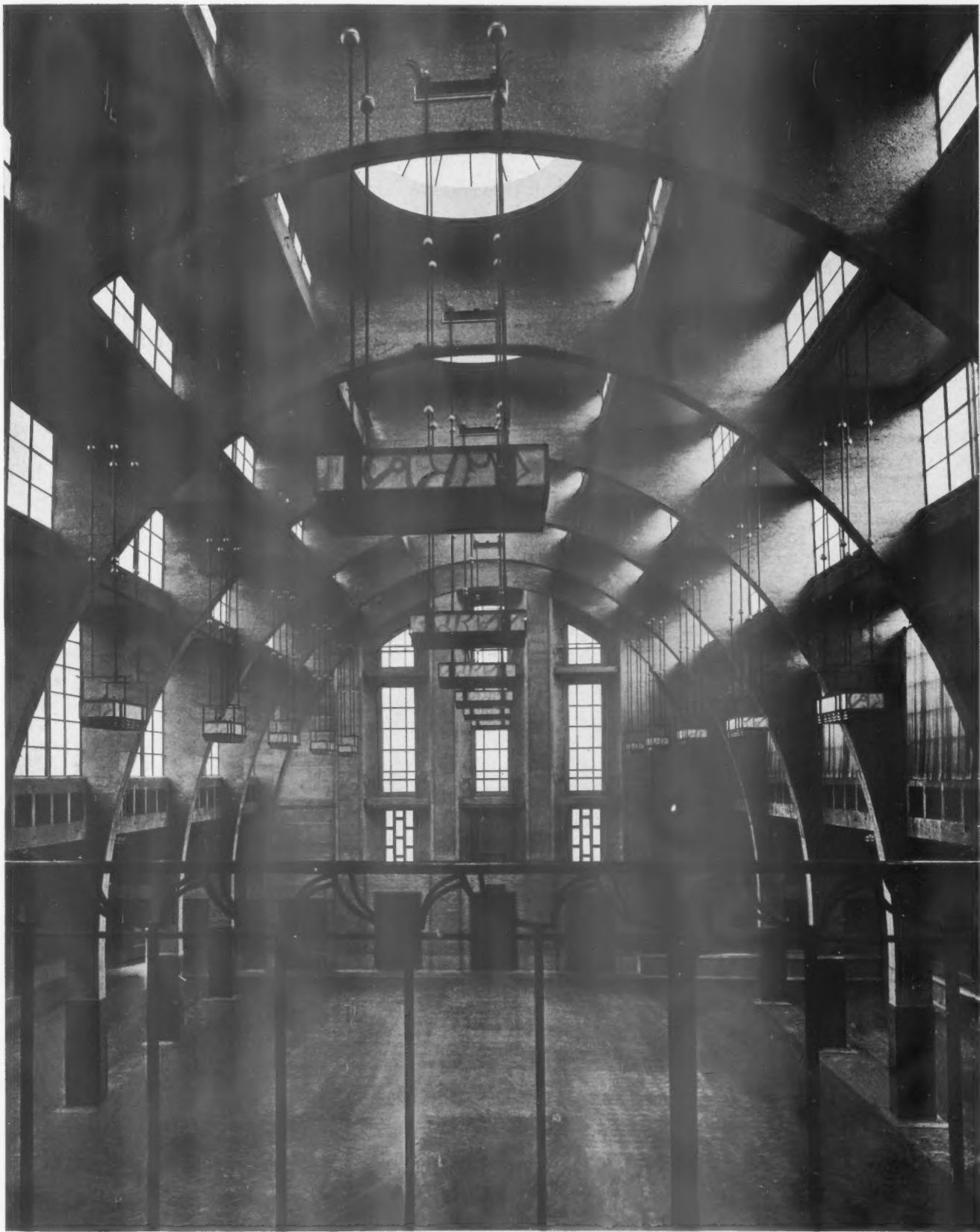
The main Exhibition HALL looking towards the EAST End. A view of the ROOF from the BALCONY .
