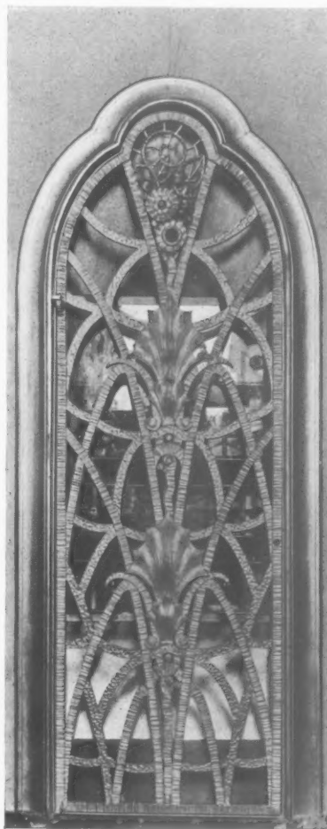
Left: The CHEVALIER grille. Made in WROUGHT and EMBOSSED IRON; the design is based on an antique grille of the Louis XIV period. Designers and Craftsmen: BAGUES.
