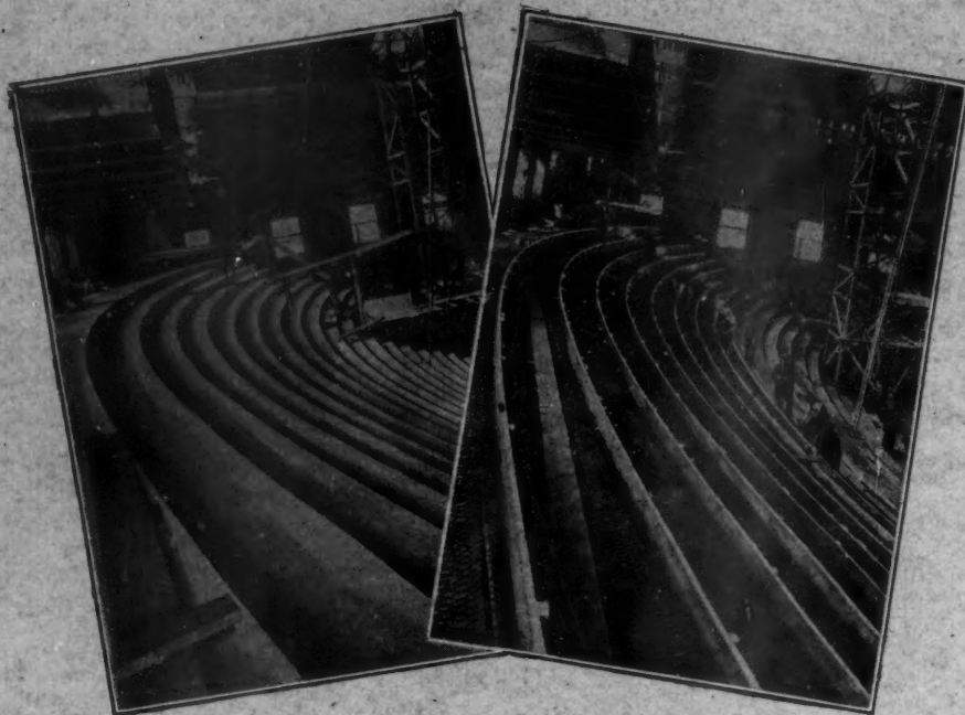
TWO STAGES OF THE WORK ON THE BALCONY On the left:—the finished work. On the right:—the laying of the reinforcement. Architects: Thos. Lamb, of New York, in collaboration with Frank Matcham & Co.
