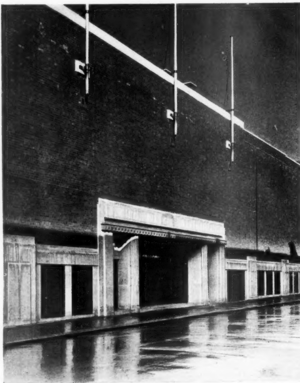
The EXIT doors in the SOUTH Front. The VALANCE on the LINTEL is of cast lead. The DOORS are made of teak, wax polished.
