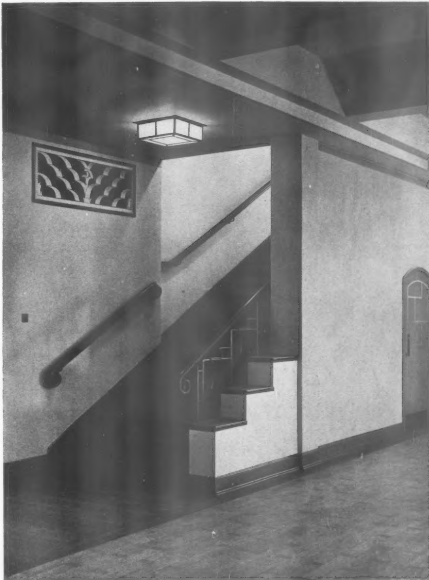
Above : The STAIRCASE in the RESTAURANT .
