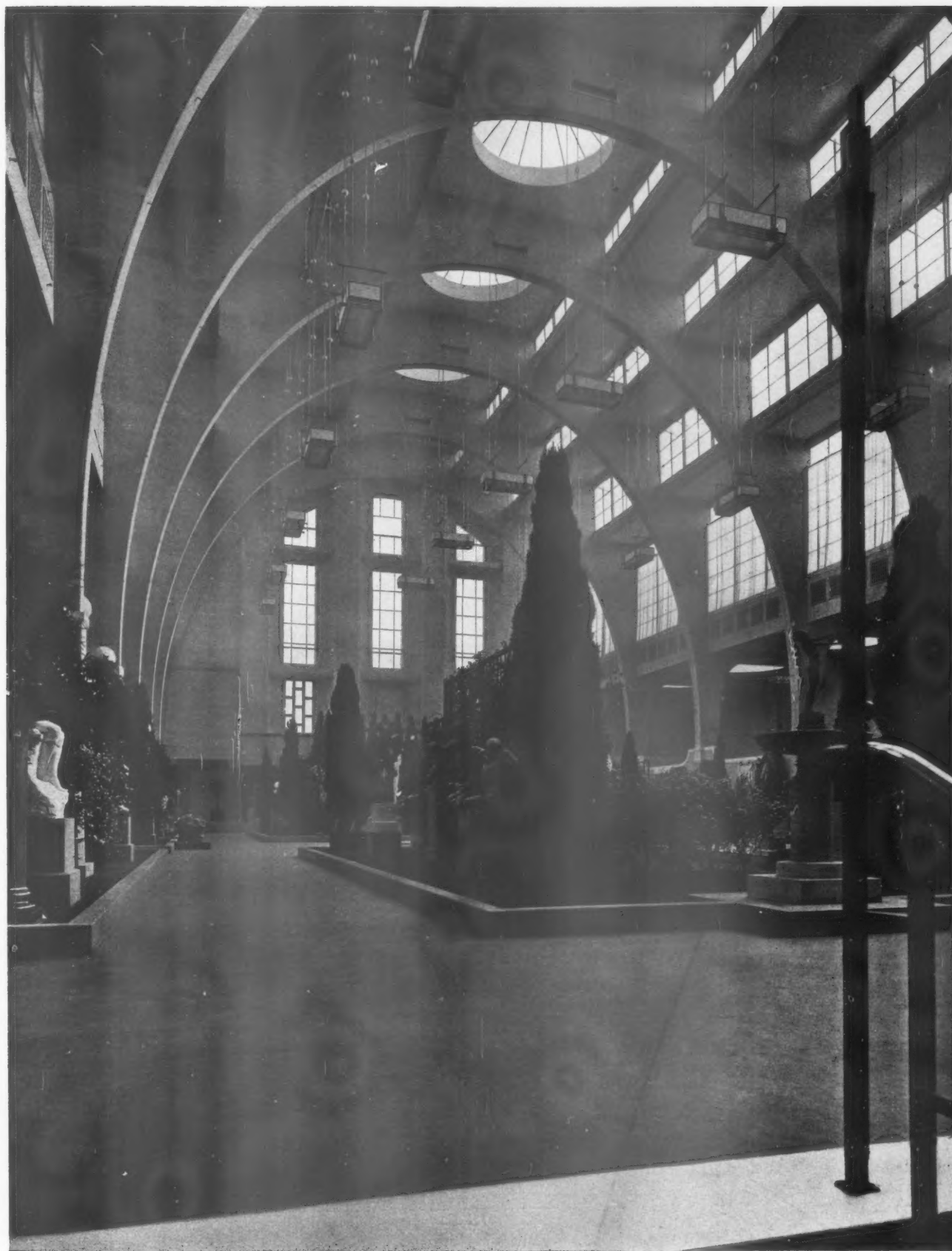
The main Exhibition HALL looking EAST from the ENTRANCE but the soffits over each tier of WINDOWS are distempered in a broken white colour. The FABRIC is built of reinforced concrete with a bush hammered face showing the grey-brown colour of the aggregate, plaster. The FLOOR is laid with pitch pine with bands of teak.
