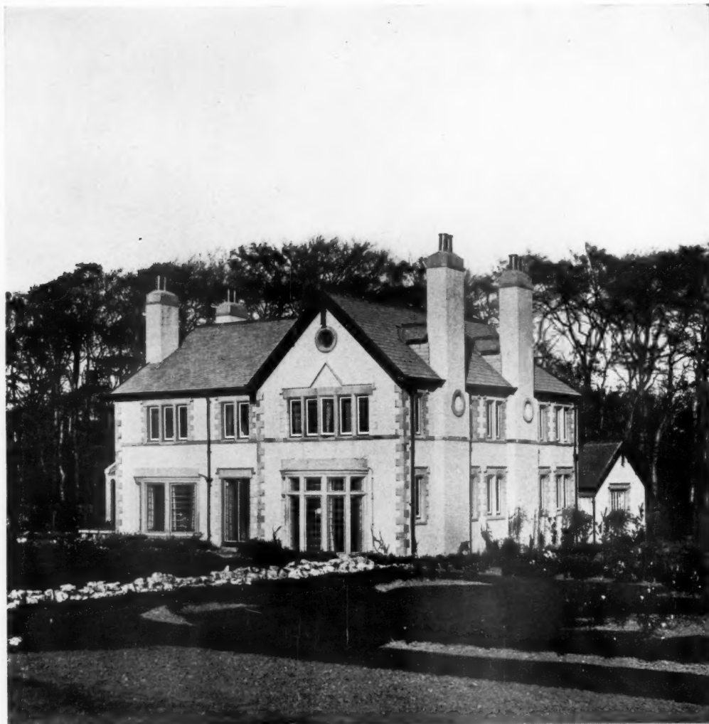
STEEL WINDOWS AND LEADED GLASS
