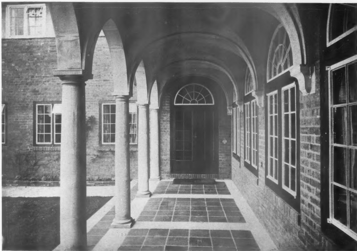
The LOGGIA on the GARDEN Side.
