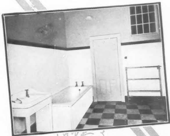
Bathroom. White and Lavender Vitrolite dado and White Vitrolite casing to bath.
