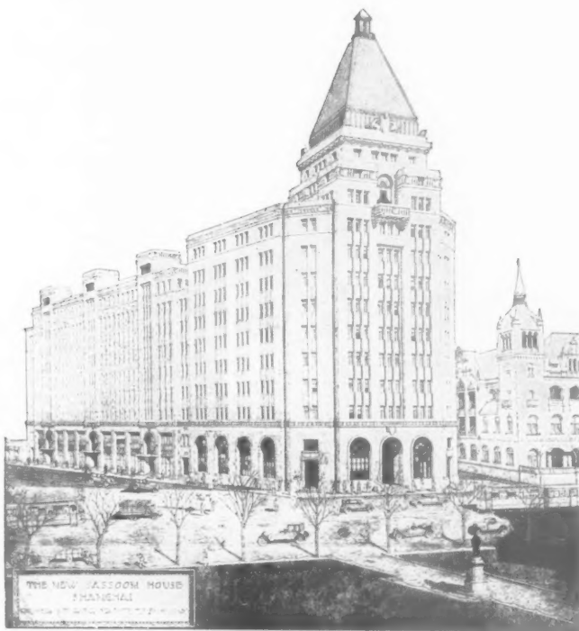
Cathay Hotel, Sassoon House, Shanghai.
