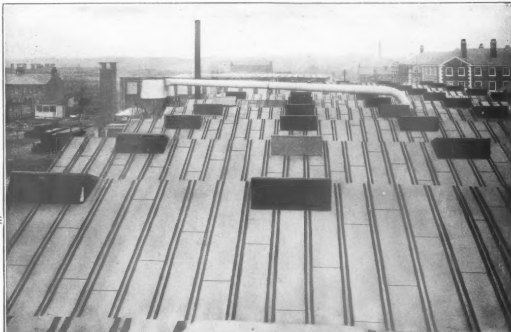
FACTORY FOR MESSRS. THE GRAMOPHONE COMPANY, LTD., HAYES, MIDDLESEX. Concrete Roof covered with Blackwells 2-ply Roofing in 1915.
