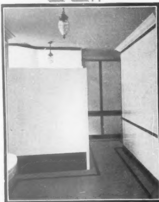
Lavatory lined with White Vitrolite Panels between Green Vitrolite skirting, dado rail and frieze.
