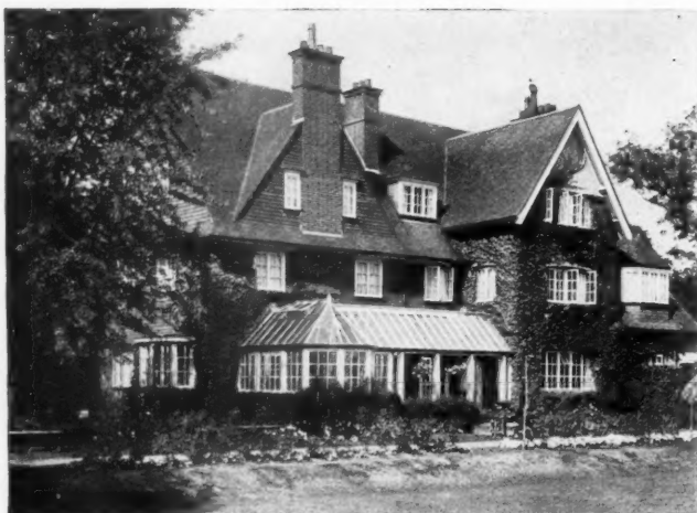
Blythswood, W. Byfleet (Residence of Sir Chas. B. Locock, Bart.) Architect : A. Burnett-Brown, Esq. Installation by Chas. P. Kinnell & Co., Ltd.
