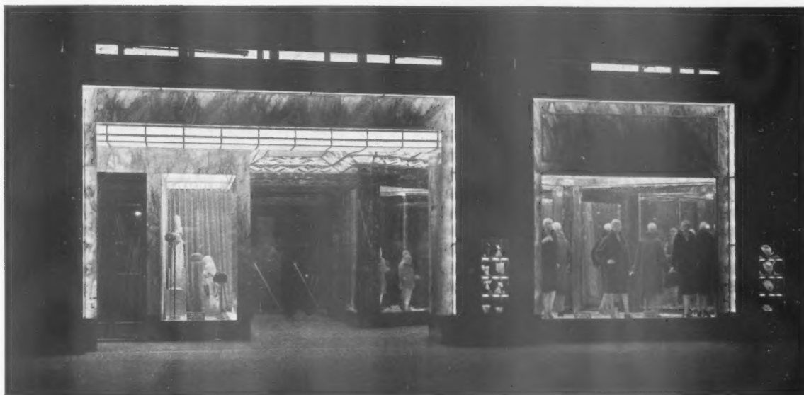
FIG. 1.—The GALLERIES LAFAYETTE, Regent Street, London.—Though Lafayette's new shop is not yet complete, enough can be seen to show that it is at present the most interesting front in London, almost the only example in England of a well-thought-out lighting scheme. The idea is roughly that of a theatre. The main front is left dark and fulfils the function of the proscenium arch. The opening is treated as a stage within which is built a second brilliantly lighted shop front with entrances set at various angles. Here the actors, who are wax models, prance and posture with a staginess entirely suitable to the conception.
