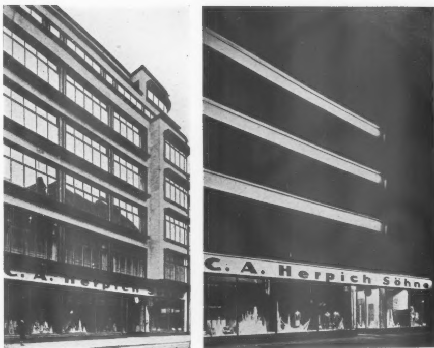
FIG. 6.—A Berlin shop by DAY and NIGHT.—The lighting is treated here in horizontal bands which, quite effective at night, are by day definitely related to the design. It is essential that schemes for night lighting should not detract from the appearance of the building by day. The best schemes are those which serve a dual purpose.
