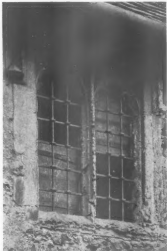
Fifteenth century. FIG. 188.—St. Cross Hospital, Winchester.
