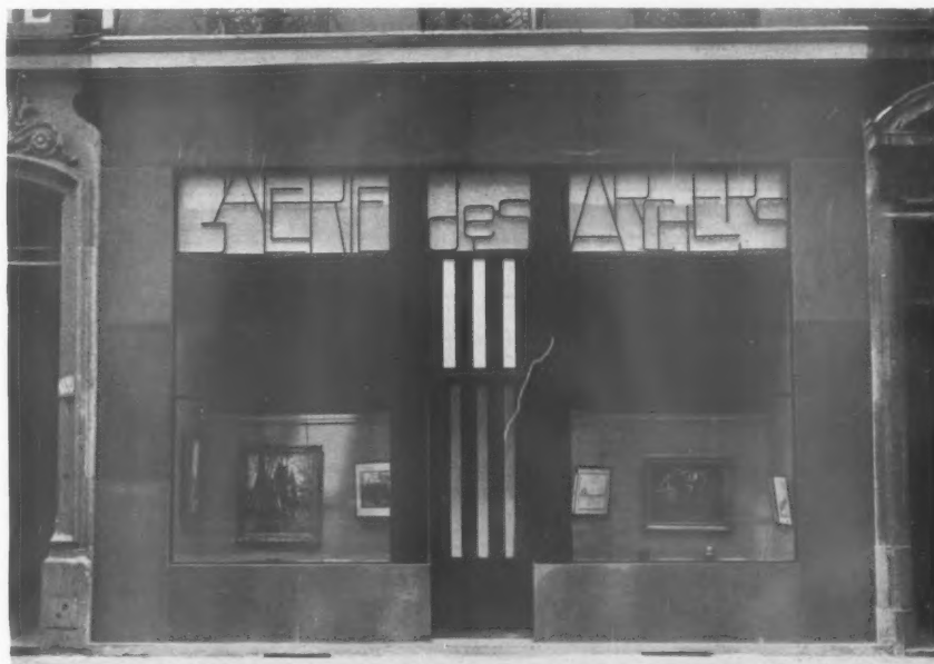
FIG. 7.—The GALERIES DES ARCHERS , Lyons. Designed by Francis Jourdain. The lettering provides the entire decorative motif for the front. This applies by night as well. The doorway and lettering are thrown in silhouette by lights behind the glass.
