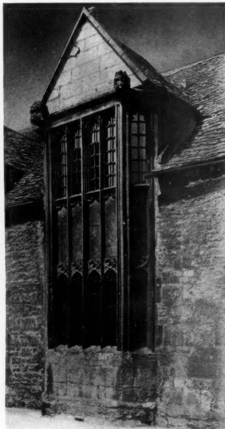
Early fifteenth century. FIG. 186.—Grevel House, Chipping Campden.
