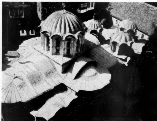
The main church at the Monastery of CHILANDARI showing the lead roofs.
