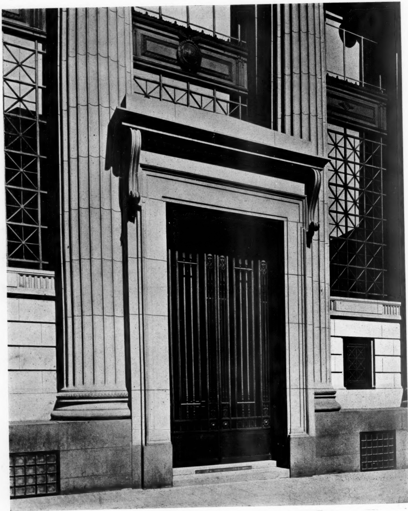
THE MAIN ENTRANCE OF THE UNION BANK OF SCOTLAND.
