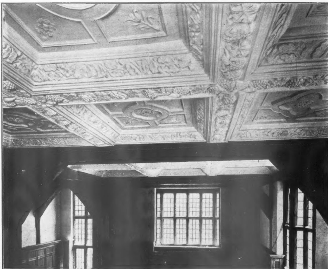
Fibrous plaster ceiling erected at the National Provincial Bank, Corwen. Architect: Capt. Ridge, A.R.I.B.A.
