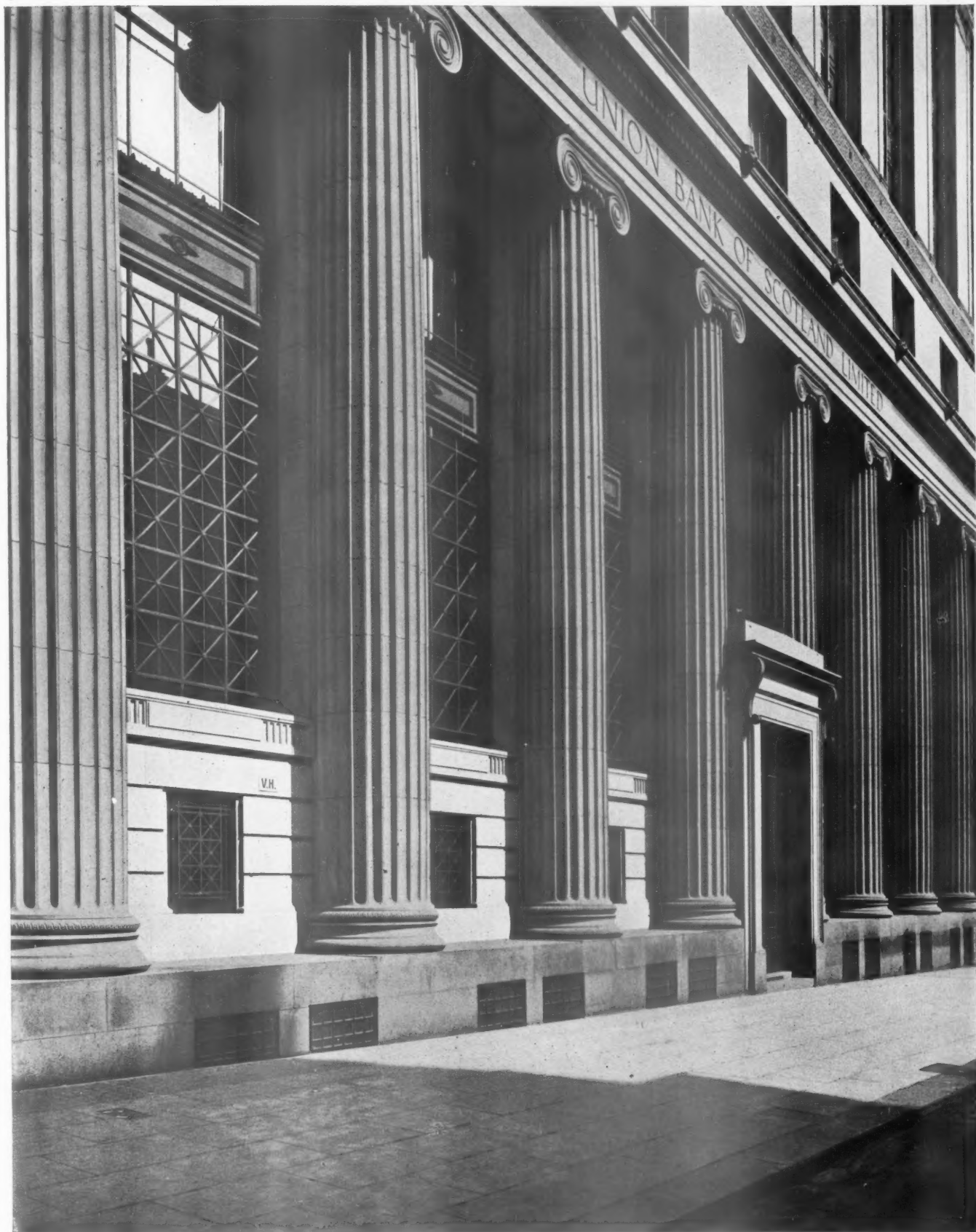
THE LOWER PART OF THE MAIN FRONT.
