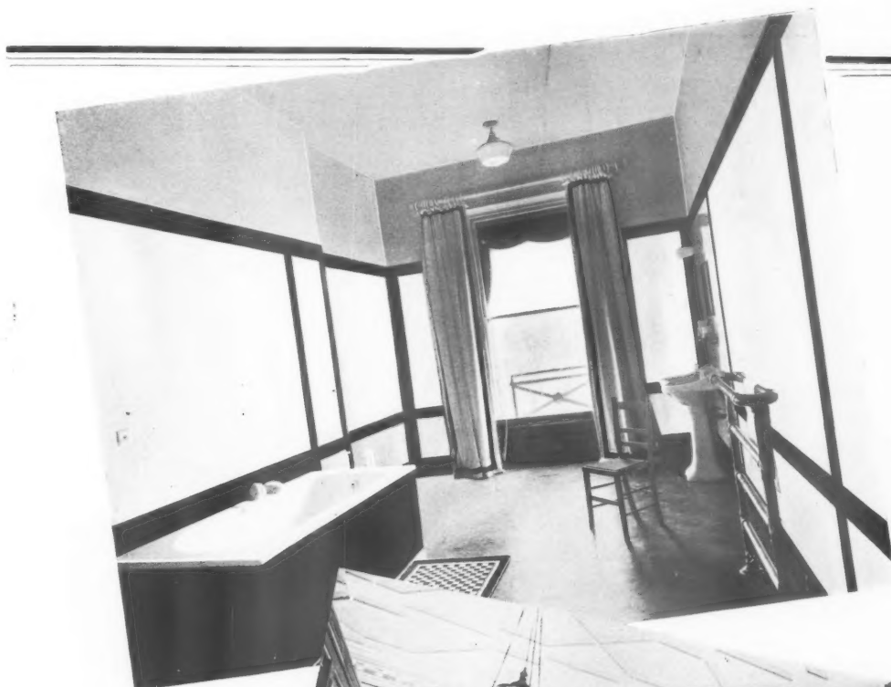
Bathroom, Private House, Hyde Park Gardens
