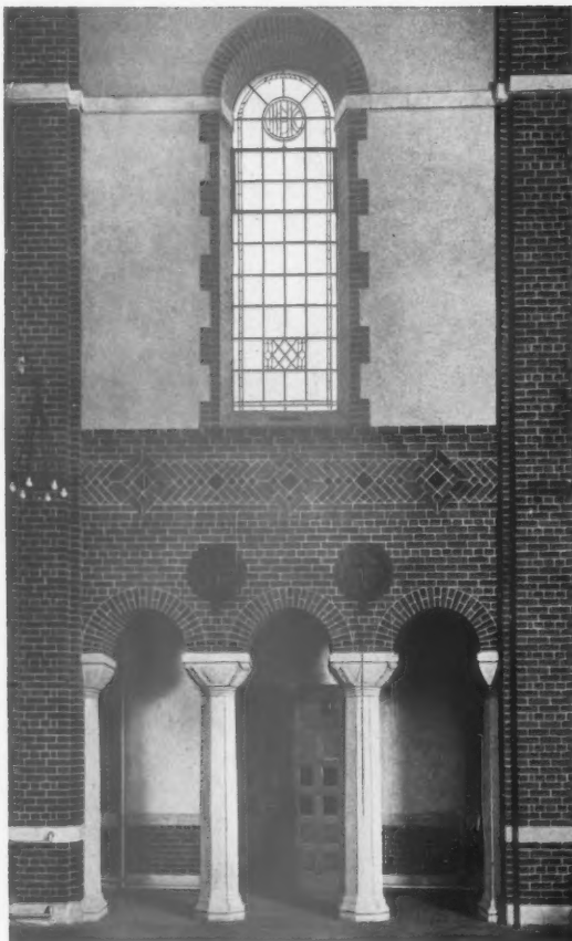
A BAY IN THE NAVE.
