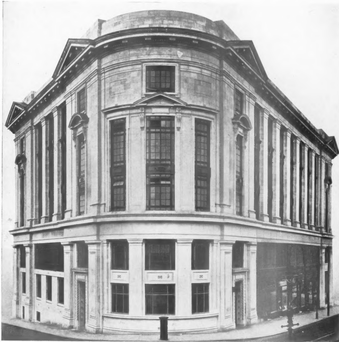
CAST IRON BUILDING FRONT AT SHEFFIELD TELEPHONE EXCHANGE. SUPPLIED AND ERECTED FOR HIS MAJESTY'S OFFICE OF WORKS BY
