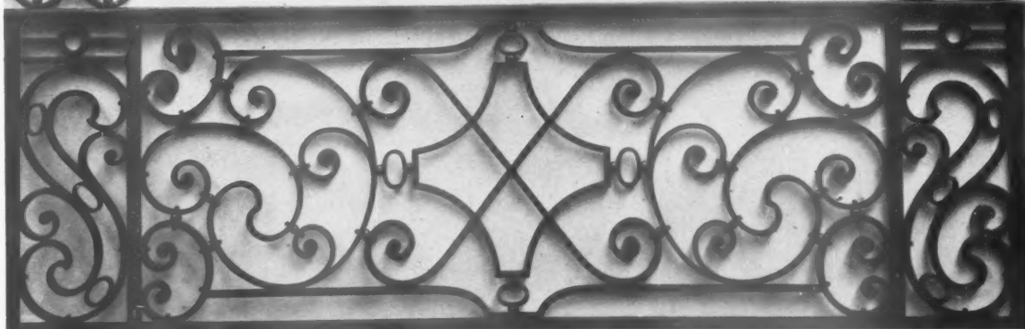
A wrought-iron balcony on the Swan and Edgar building. The cast-iron finials are in the form of baskets of fruit.
