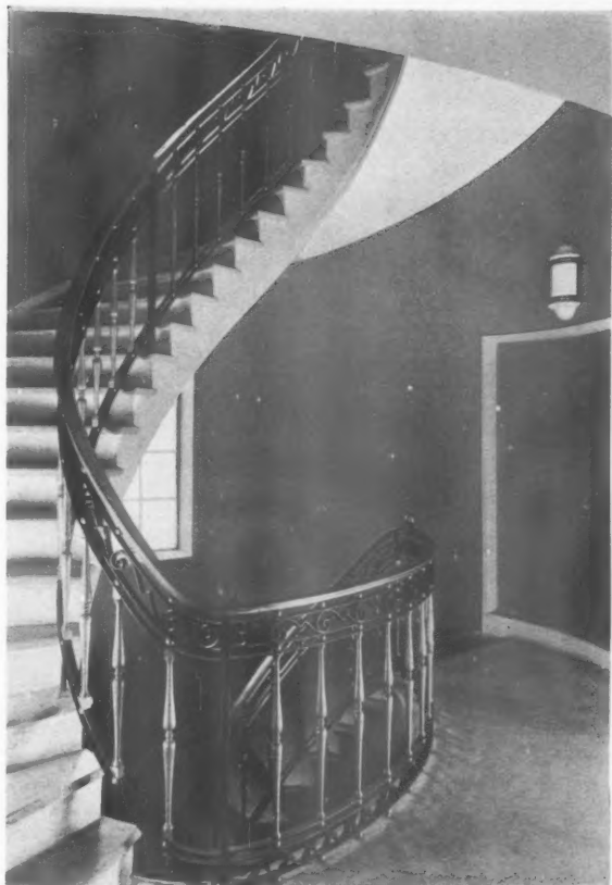
THE OVAL STAIRCASE. The balustrade is bronze and wrought-iron, and the walls are painted old rose colour.
