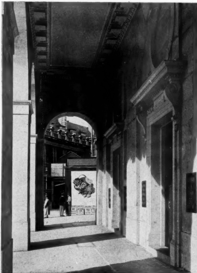
The arcade of the new County Fire Office: the last relic of Nash's great "colonnaded piazza."
