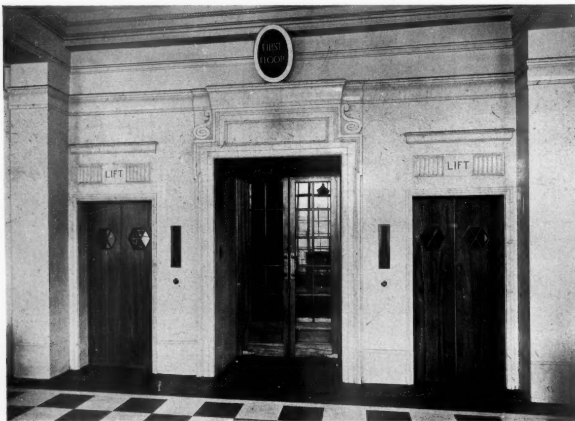
THE ENTRANCE DOORWAY AND LIFTS OF THE MAIN OFFICE ON THE FIRST FLOOR.
