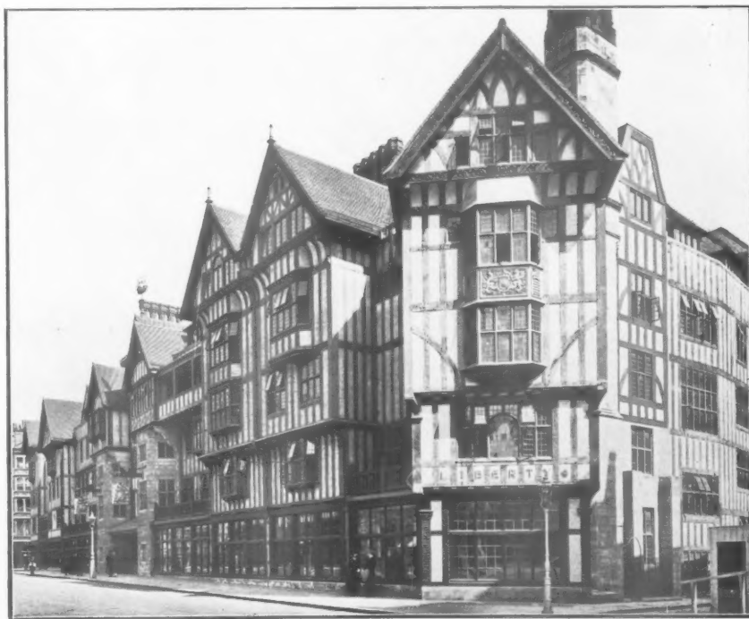
MESSRS. LIBERTY'S TUDOR BUILDING.
