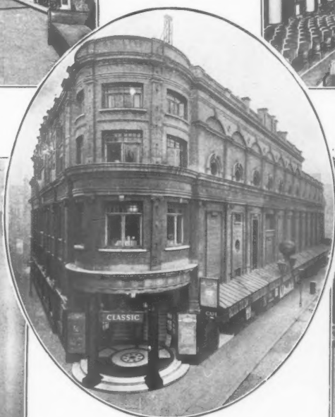
CLASSIC CINEMA, BELFAST. Architects: S. Stevenson & Sons, Belfast.
