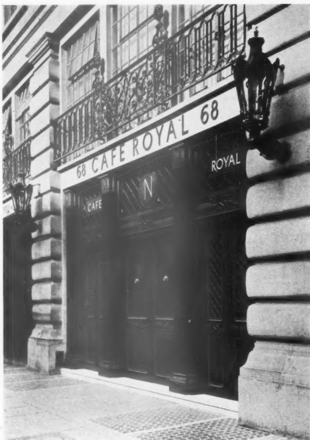
3. "On the east side of the quadrant stands the Café Royal, a dignified design which, like several other shops, finds a little difficulty in dealing with the rather meagre fascia-cum-lintel which marks the separation of street-floor and mezzanine."
