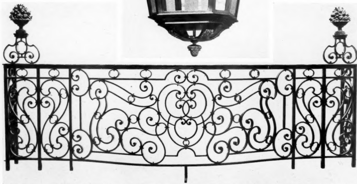
One of the five wrought-iron balconies at the County Fire Office, each measuring 12 ft. long, 3 ft. 6 in. high, and 3 ft. wide. Architect: SIR REGINALD BLOMFIELD, R.A.
