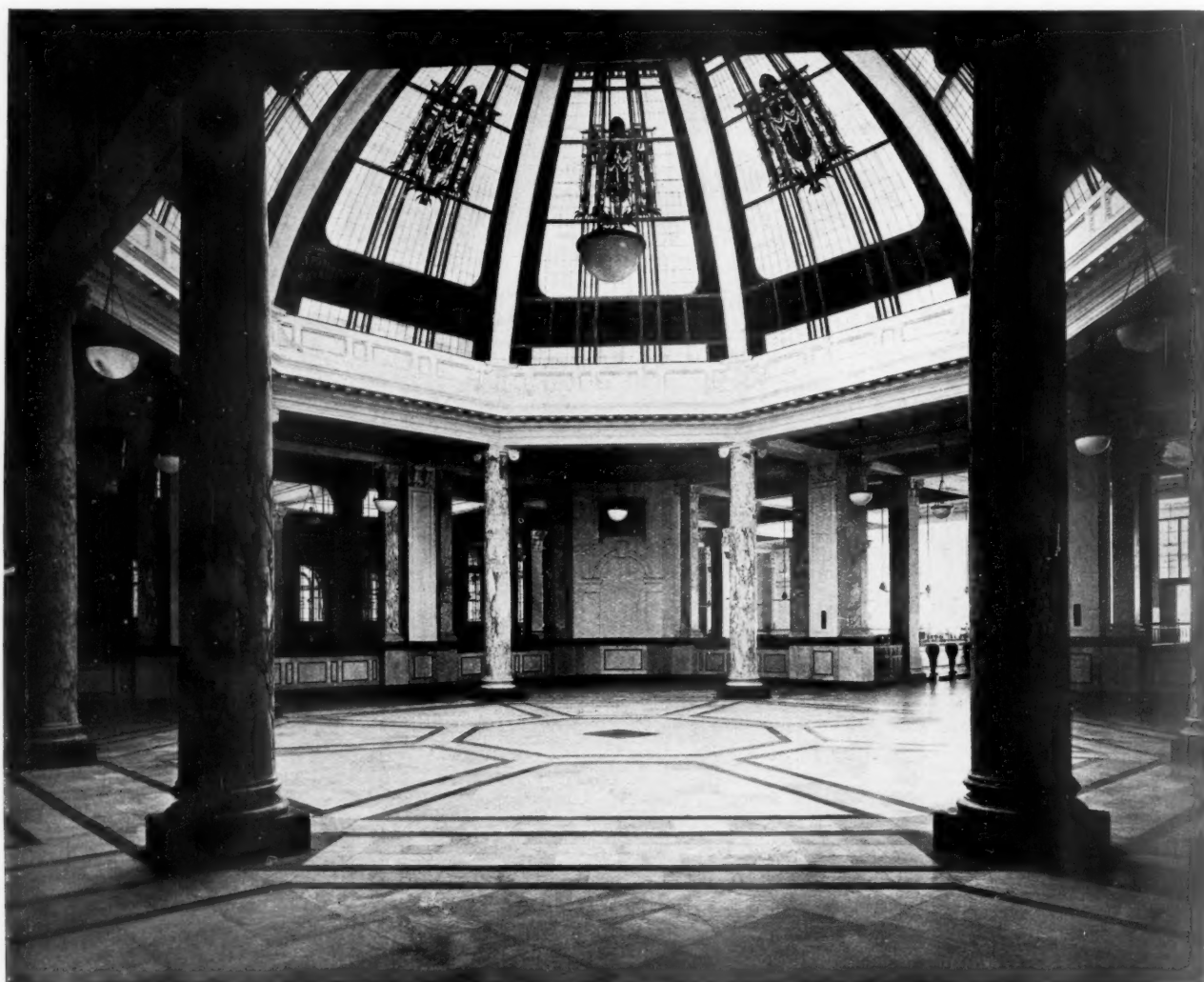
New Offices, Strand Road, Calcutta.
