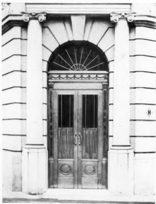
MESSRS. RIMMEL, No. 167 REGENT STREET SILVER BRONZE DOORS. ALSO SHOP FRONTS WITH SYCAMORE SHOWCASES BEHIND.
