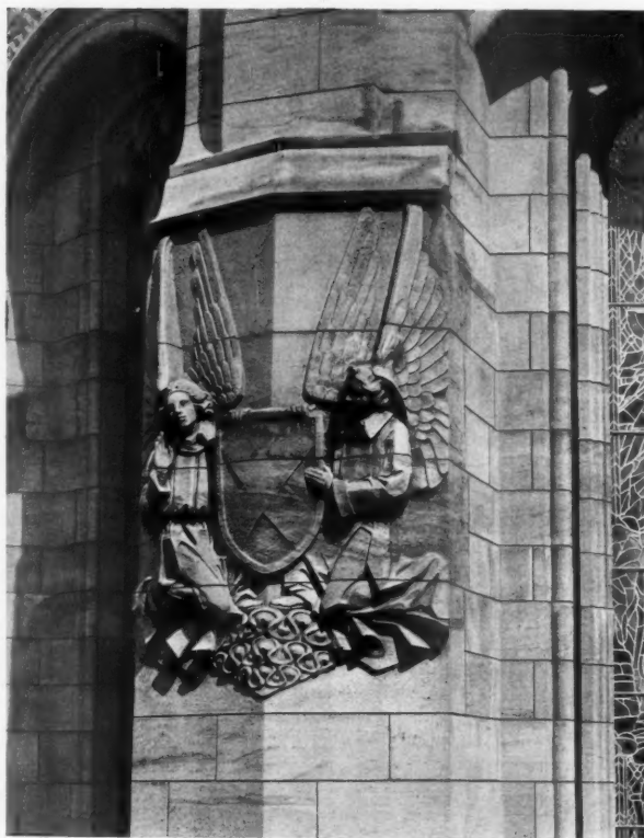
Carved angels supporting the Cross of St. Andrew on one of the buttresses of the Shrine.
