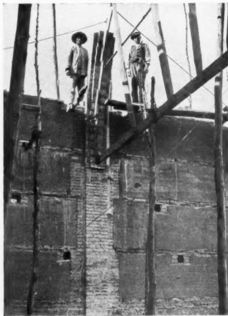
10. A detail of the bodega. The walls between each arch are of rammed earth ( tapia ).
