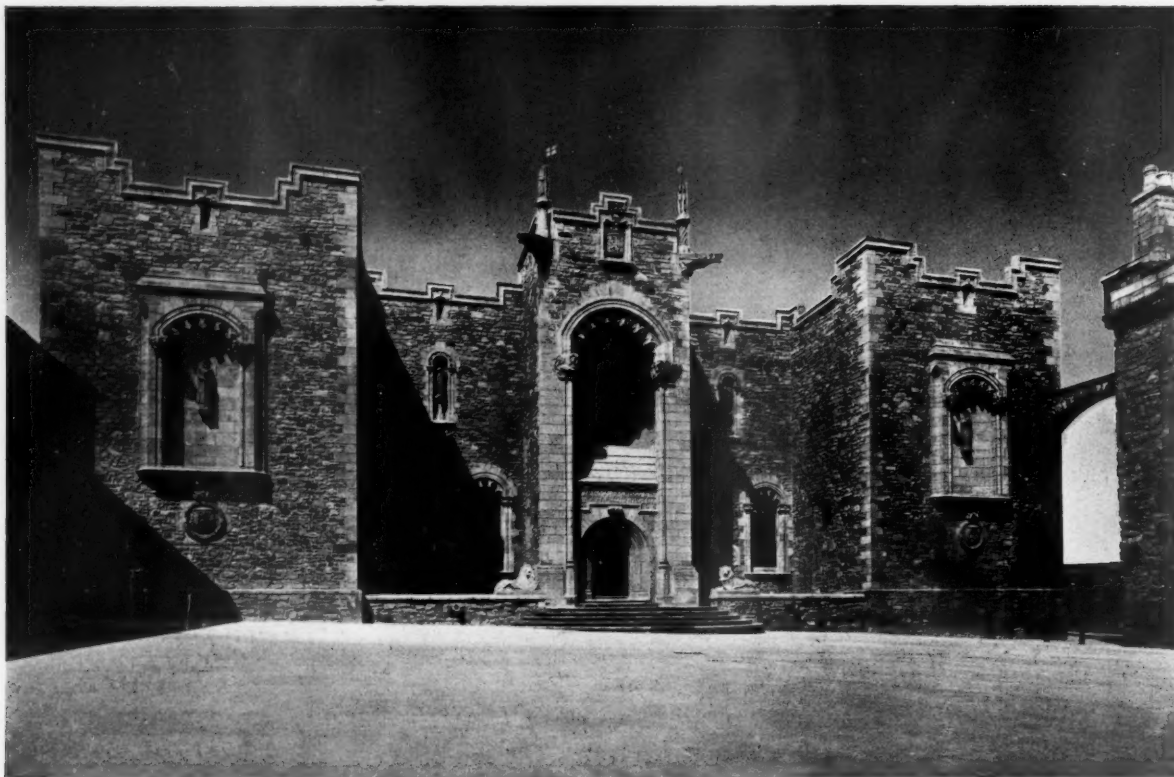
The south front facing Crown Square. In the shadow of the great arch over the entrance doorway can be seen a sculptured figure which is intended to represent the survival of the spirit.
