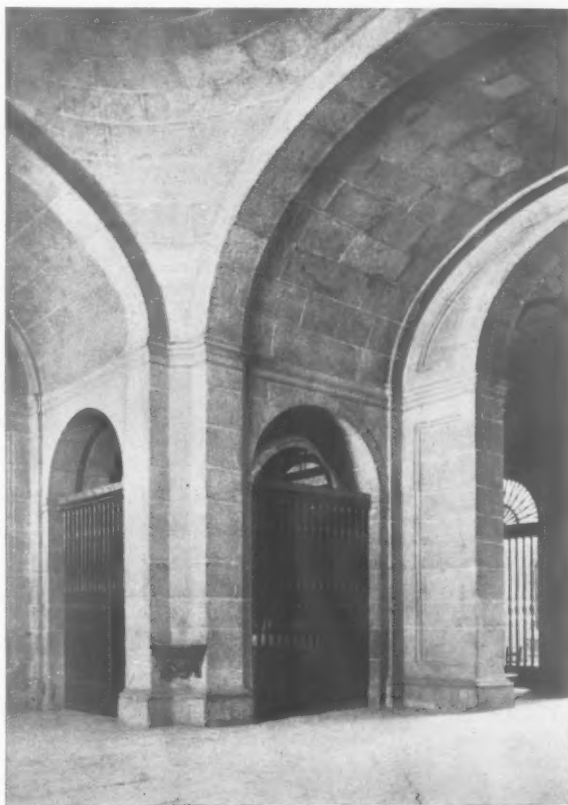
3. Granite vaulting under the Escorial choir designed by Herrera, shown here for comparison with the bridge. The saucer vault can just be seen on the left hand side.
