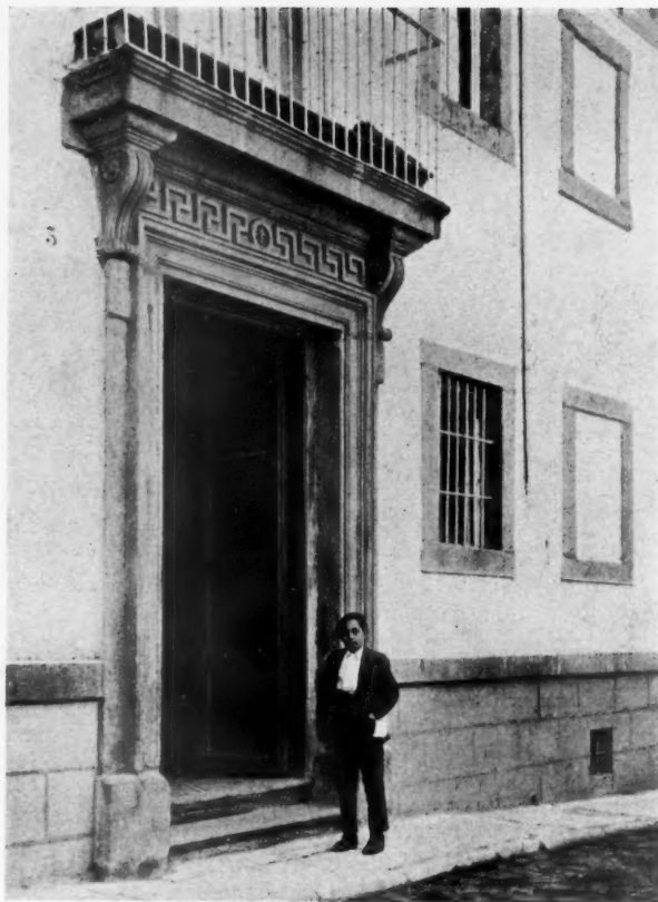
5. The House of the Queen, El Escorial, which is typical of the old granite houses in the village.
