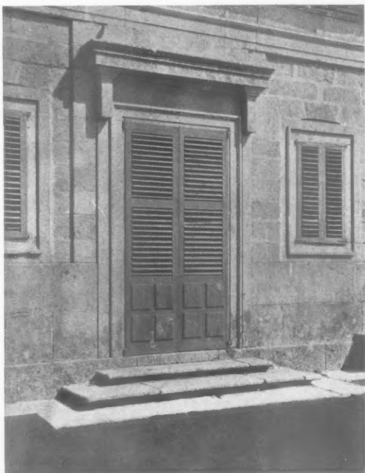
3. A side doorway to the Casita de Arriba, designed in Herrera's manner, but in a lighter vein, suited to a royal hunting lodge.
