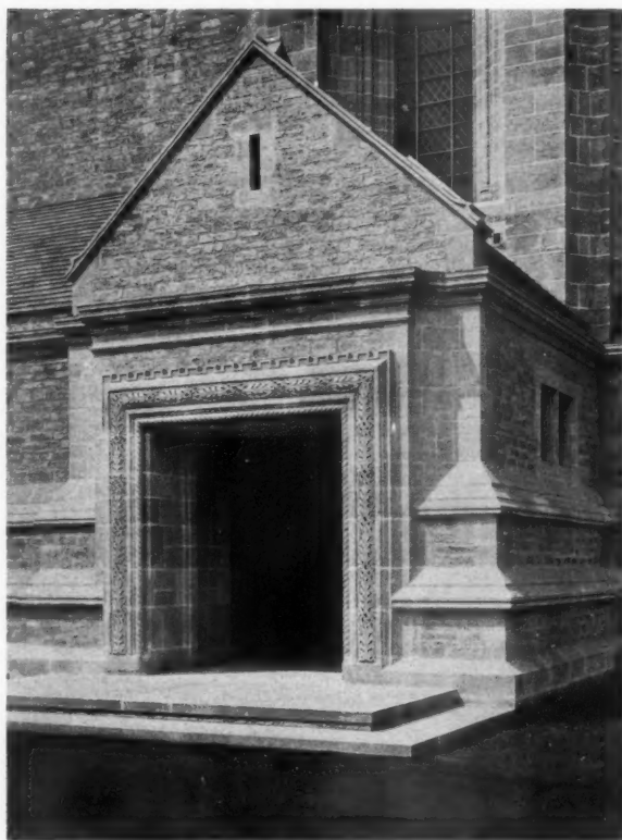
Charterhouse War Memorial School Chapel. The south-west porch.
