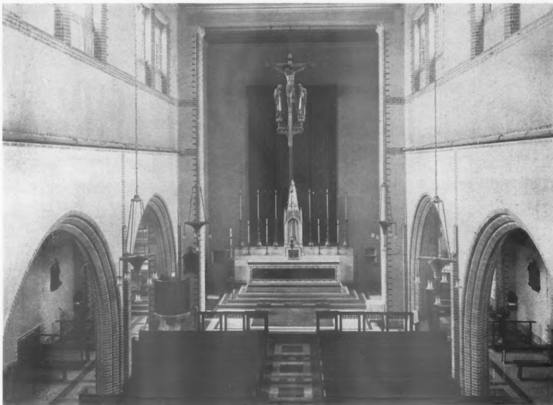
THE NAVE OF THE CHURCH OF OUR LADY, NORTHFLEET, KENT. Sir Giles Gilbert Scott, R.A., Architect.
