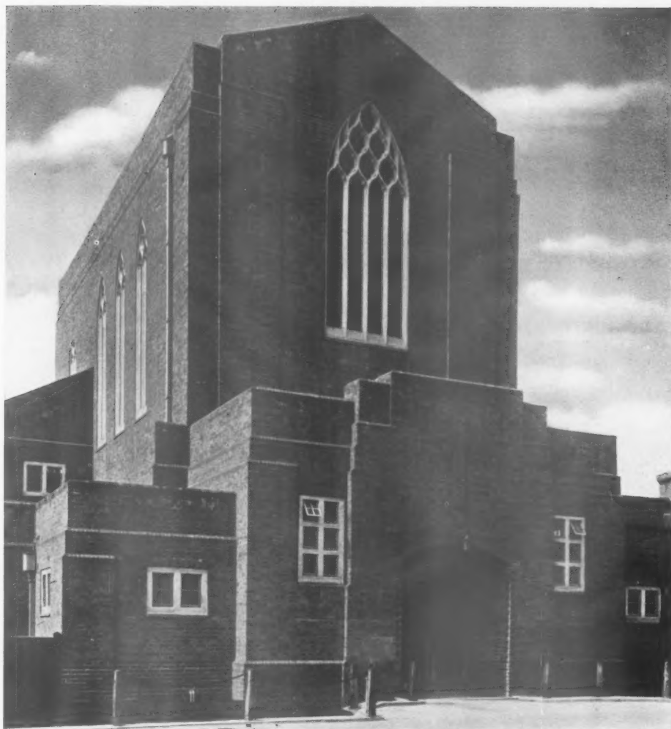
ST. SAVIOUR'S CHURCH, ACTON. THE WEST END. Edward Maufe, Architect.
