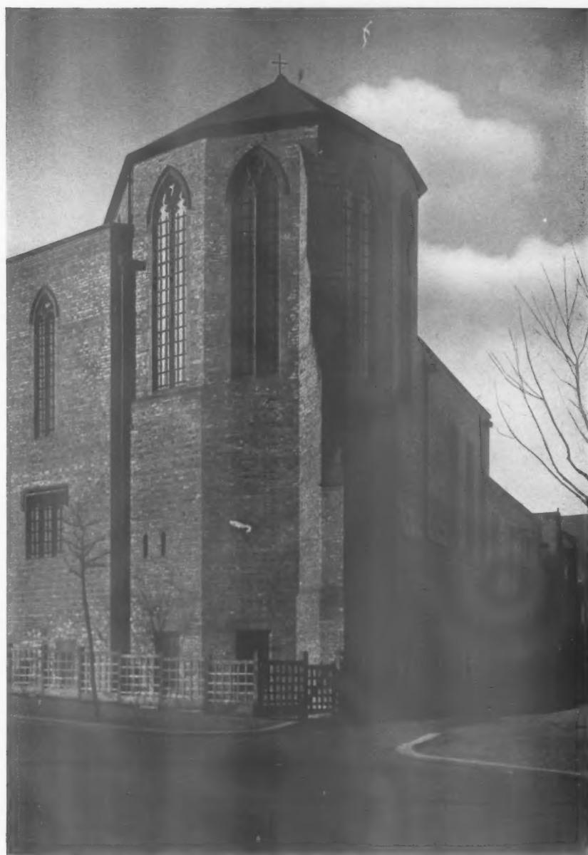
THE APSE OF THE CHURCH OF ST. COLUMBA, SCARBOROUGH. Temple Moore and Moore, Architects.
