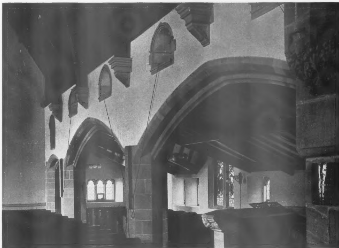
THE NEW NORTH WALL AND AISLE IN WILLASTON CHURCH, CHESHIRE. Bernard Miller, Architect.
