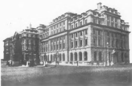
North British and Mercantile Insurance Co., and Lloyds Bank, Waterloo Place.
