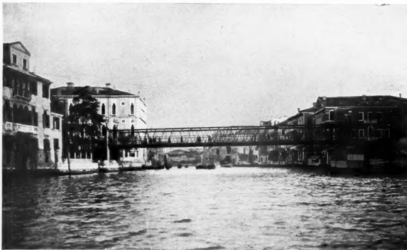
The old iron bridge.
