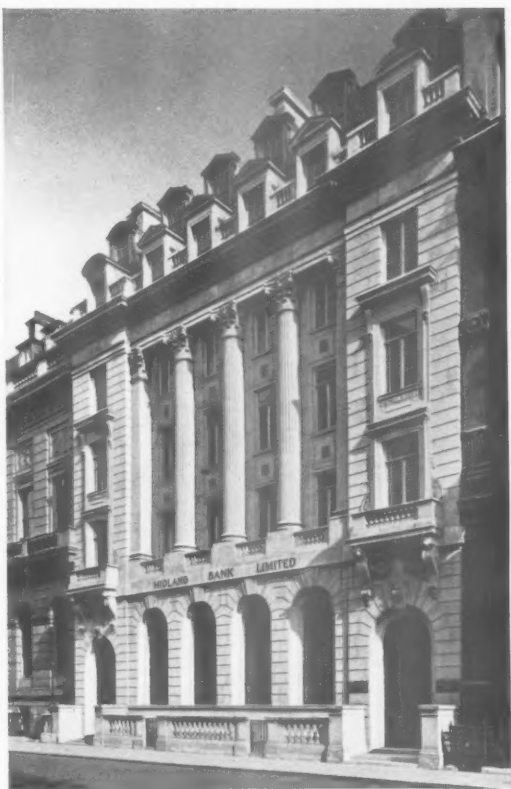
THE MIDLAND BANK, PALL MALL. Architects: Messrs Whinney, Son, and Austen Hall.
