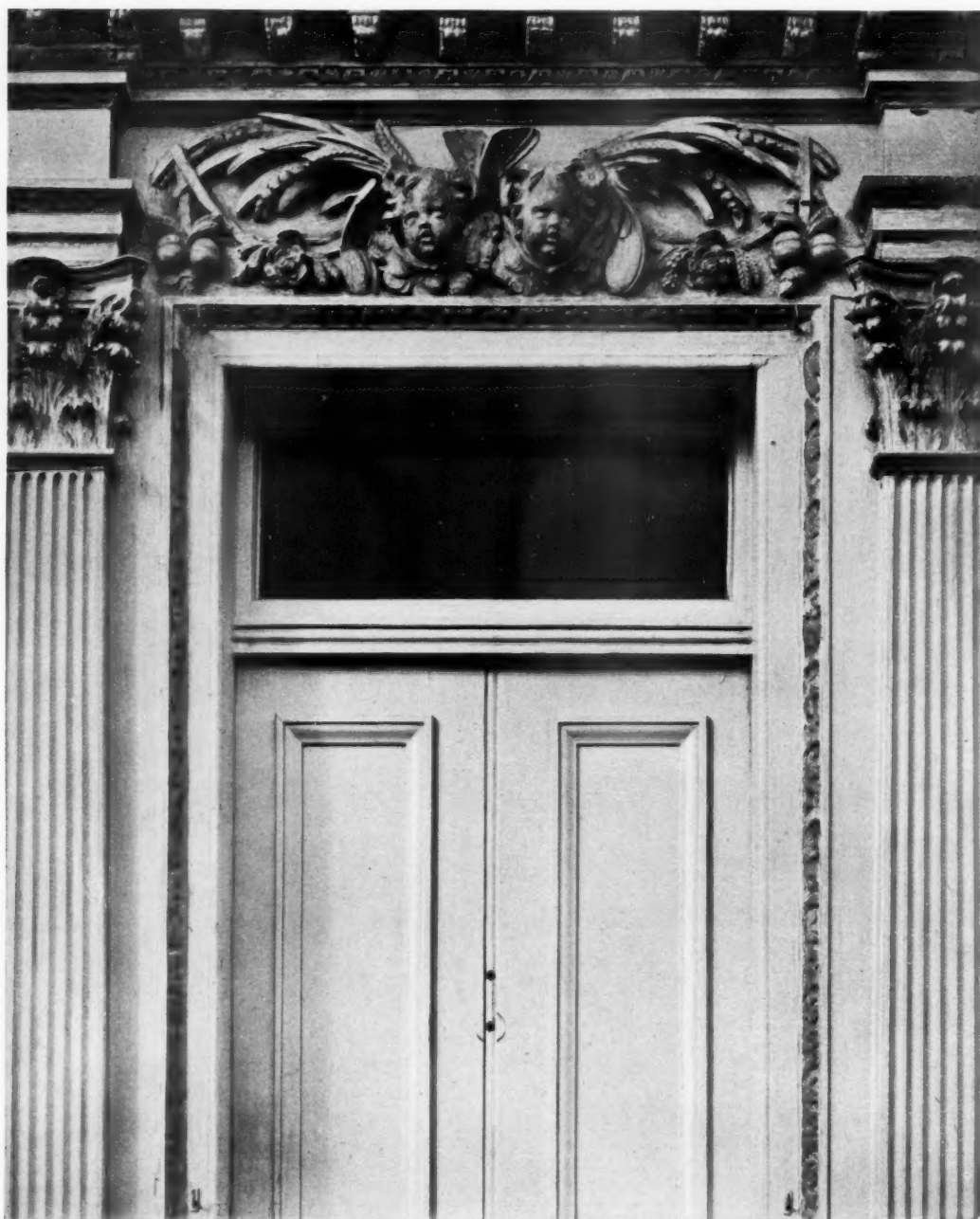
A DETAIL OF THE FRONT DOOR CASE.
