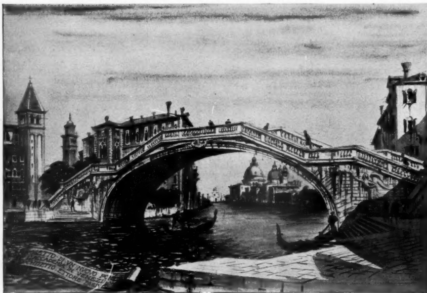
The new bridge.
