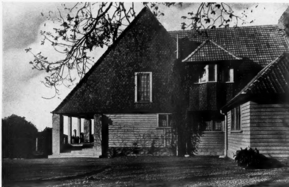
"Fairley," Auckland, the residence of A. McCosh Clark, Esq. The house from the forecourt. The walls are built of Kauri weather-boarding from a stone base to a height of 7 ft. 6 in., and painted grey. The upper portion is covered with shingles left to weather, which have toned to a mellow blend of greys and greens.
