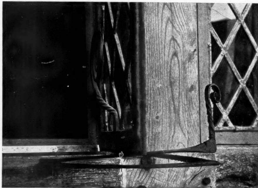
FIG. 8. A QUADRANT WITH A VOLUTED TERMINAL.
