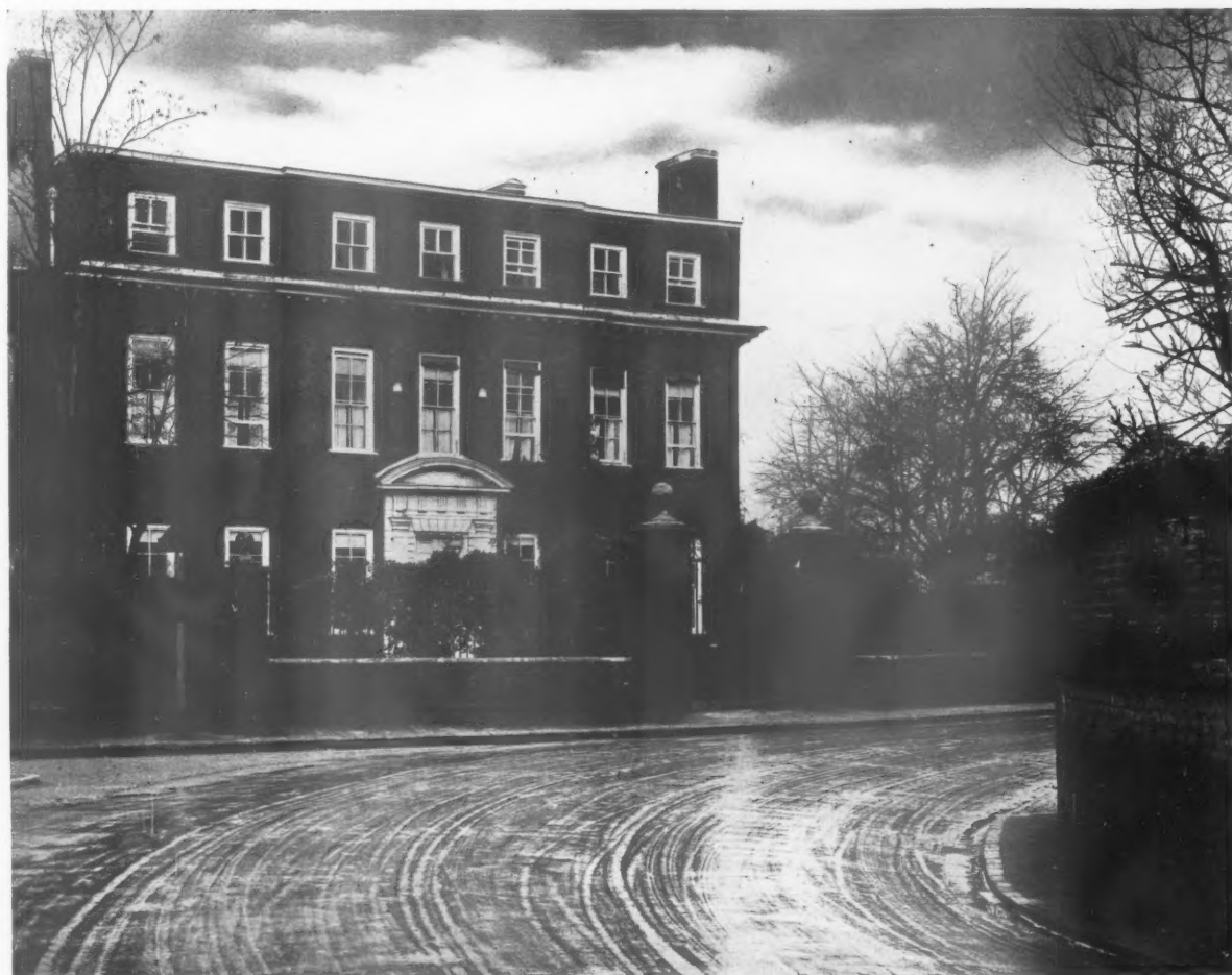
THE HOUSE FROM THE ROAD.
