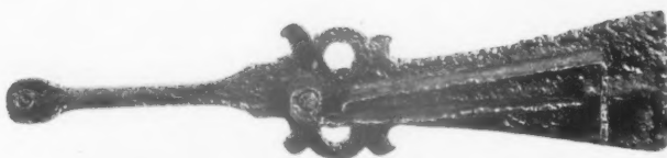
FIG. 5. ENGLISH CASEMENT-LATCHES OF THE SIXTEENTH AND SEVENTEENTH CENTURIES.
