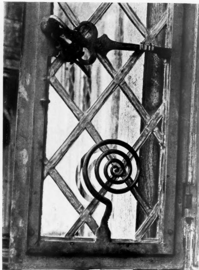
FIG. 7. A VOLUTED HANDLE, AND A MODERN TURNIL, PLATE AND BAR BASED ON AN OLD DESIGN.
