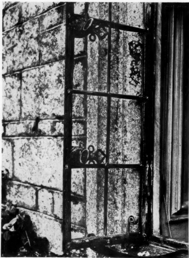
FIG. 6. A CASEMENT WITH TWO TURNILS AND PLATES, A HANDLE FOR DRAWING THE CASEMENT IN, AND A QUADRANT.
