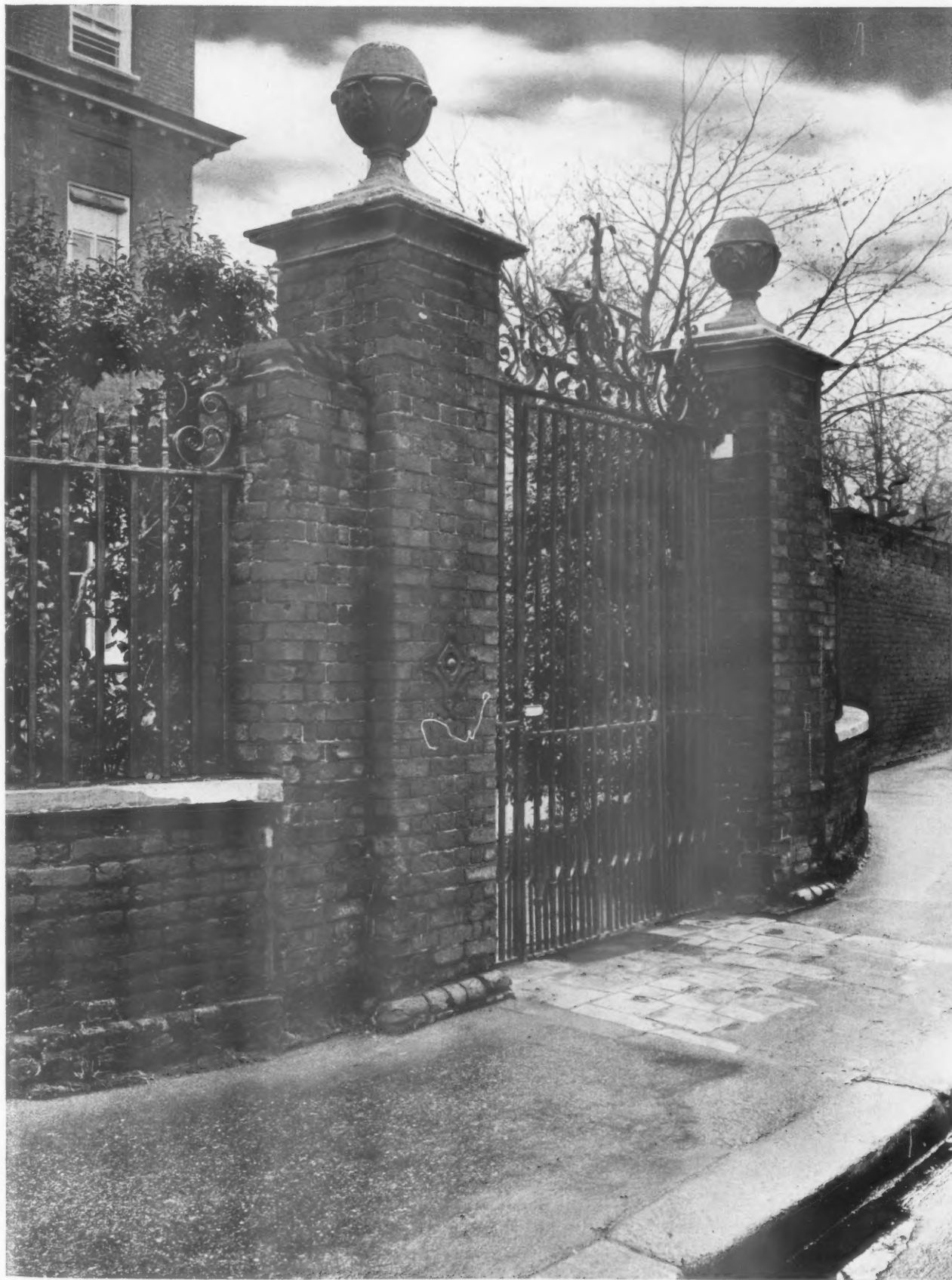
THE ENTRANCE GATES.
