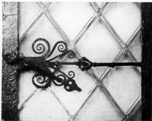
FIG. 3. A CASEMENT-LATCH.
