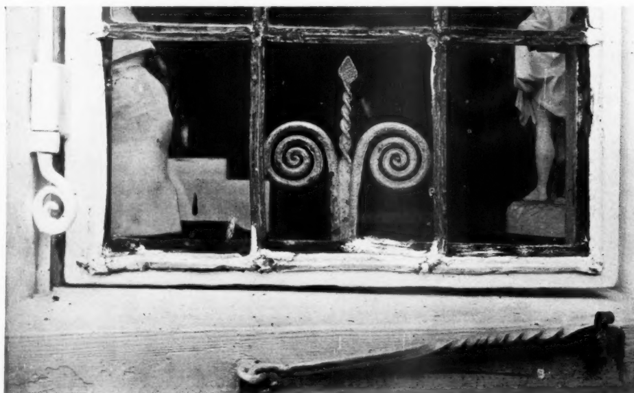
FIG. 12. A HANDLE, HINGE TERMINAL, AND OLD-FASHIONED HOOK STAY.
