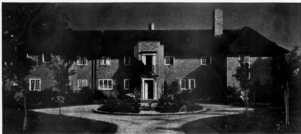
THE MAIN FRONT AND THE FORECOURT.
