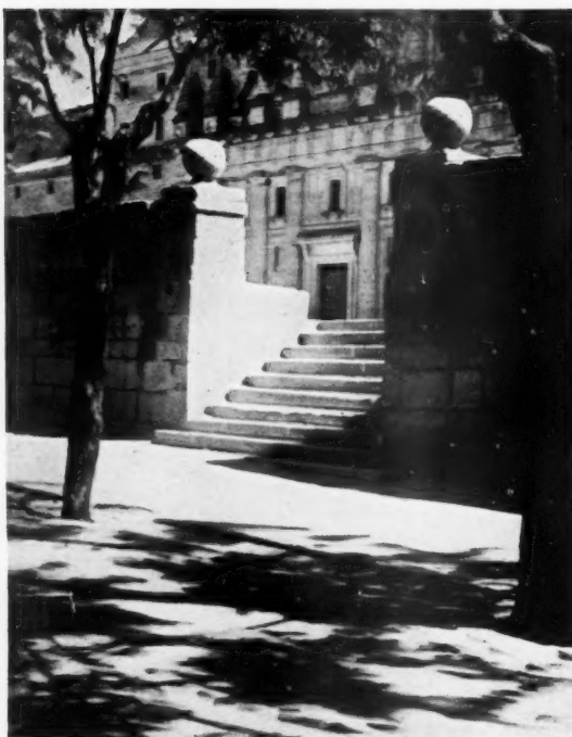
1. Steps leading to the main entrance.
