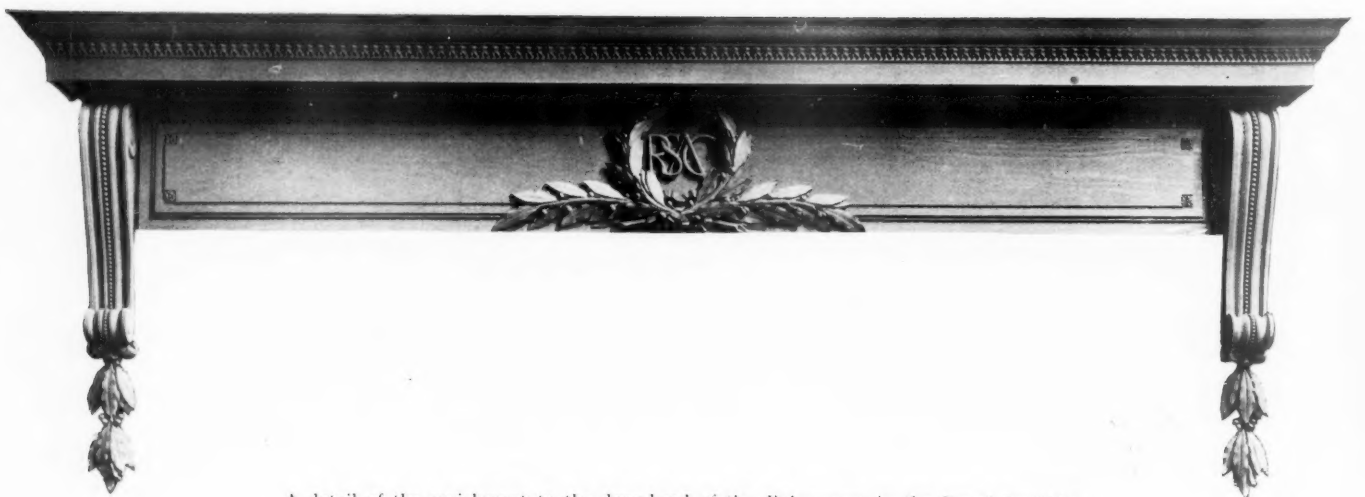
A detail of the enrichment to the door head of the dining-room in the Royal Scottish Automobile Club, Glasgow.
