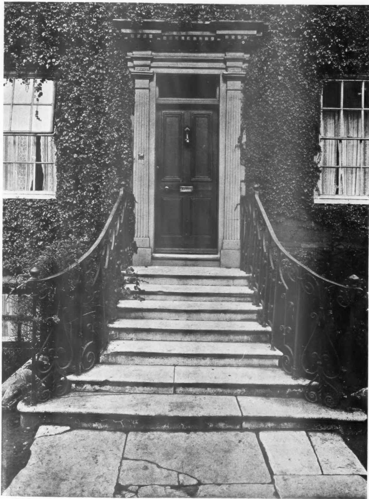
THE ENTRANCE DOORWAY.
