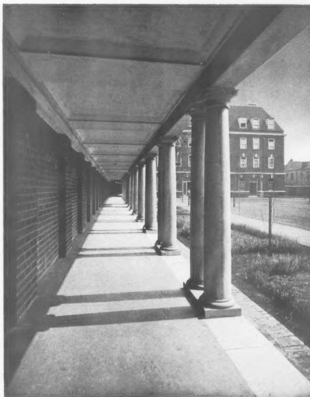
THE COVERED-WAY CONNECTING THE TWO BUILDINGS.
