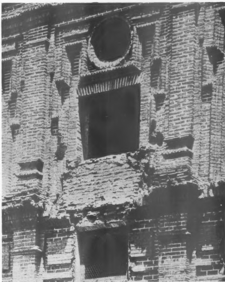
6. A WINDOW IN THE PATIO, LA MERCED, CALATAYUD.
