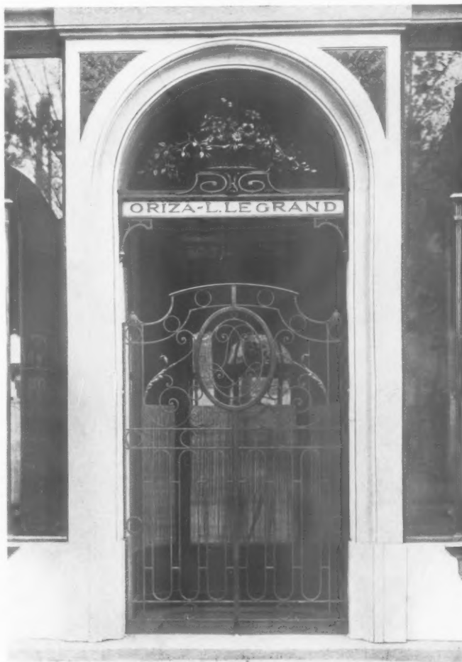
A DETAIL OF THE IRONWORK IN ORIZA-LEGRAND'S SHOP.
