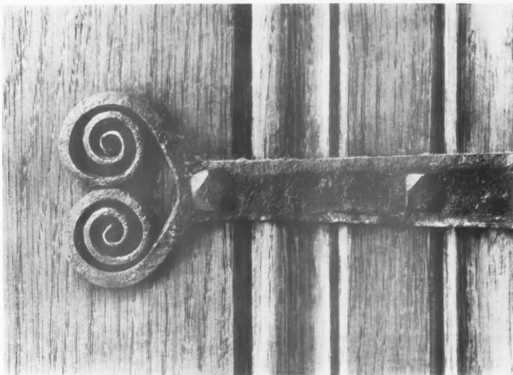
4. THE CHAMFERED STRAP.
