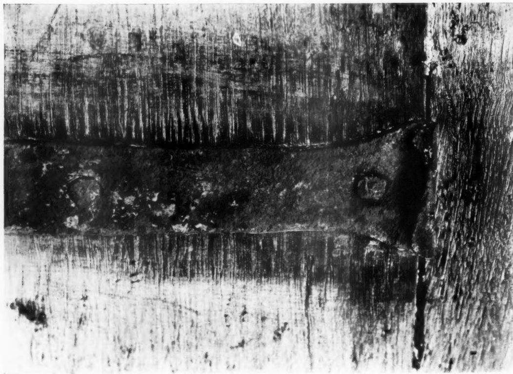
2. TAPERED IRON HINGE.
