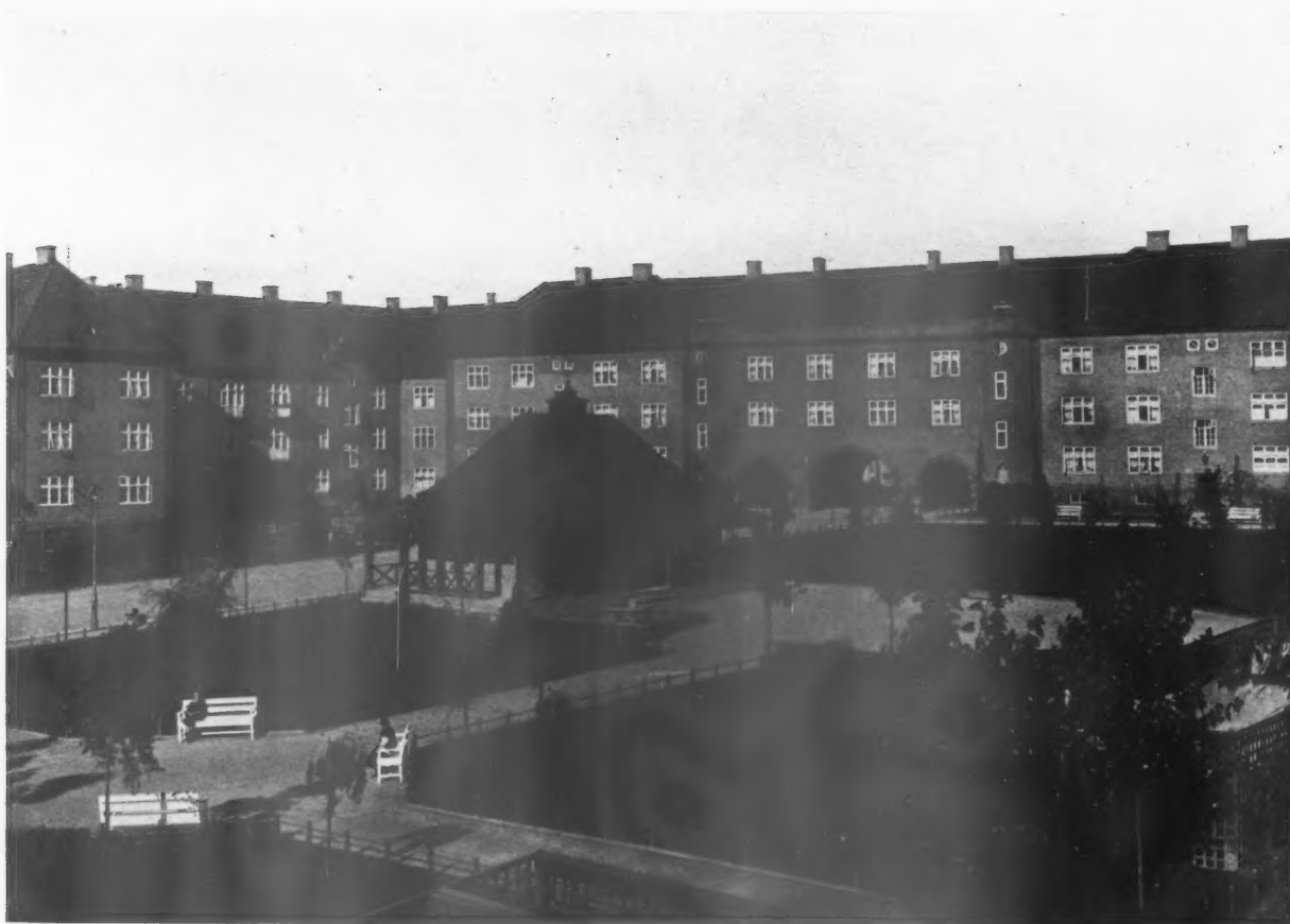
THE TORSHOV COMPLEX. THE GARDENS.
