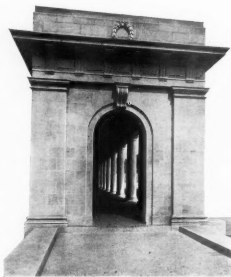
THE ENTRANCE TO THE COLONNADE.
