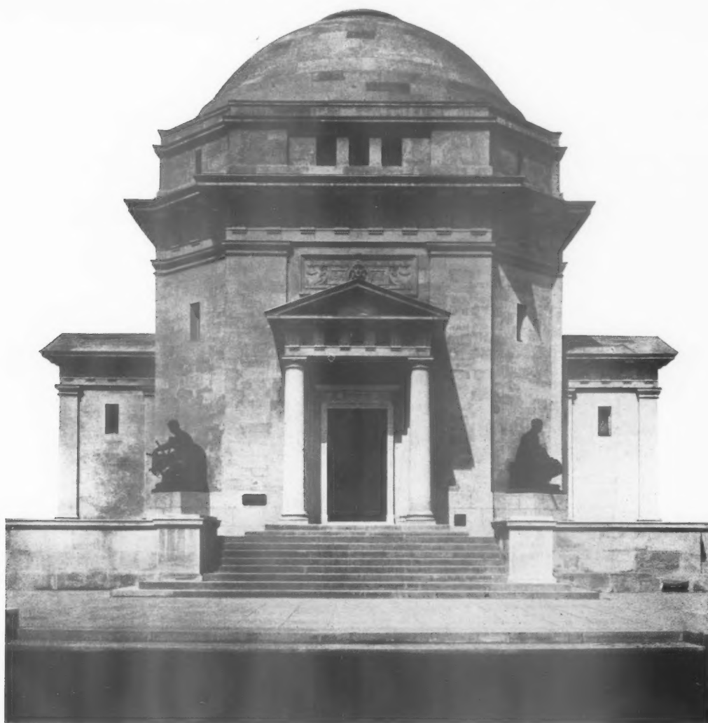
THE MAIN ENTRANCE FRONT.
