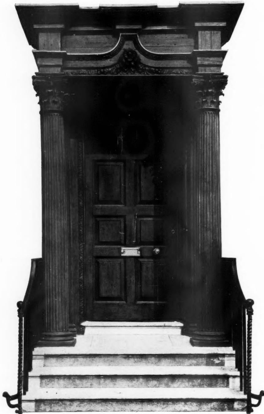
THE FRONT DOOR AND DOORCASE.
