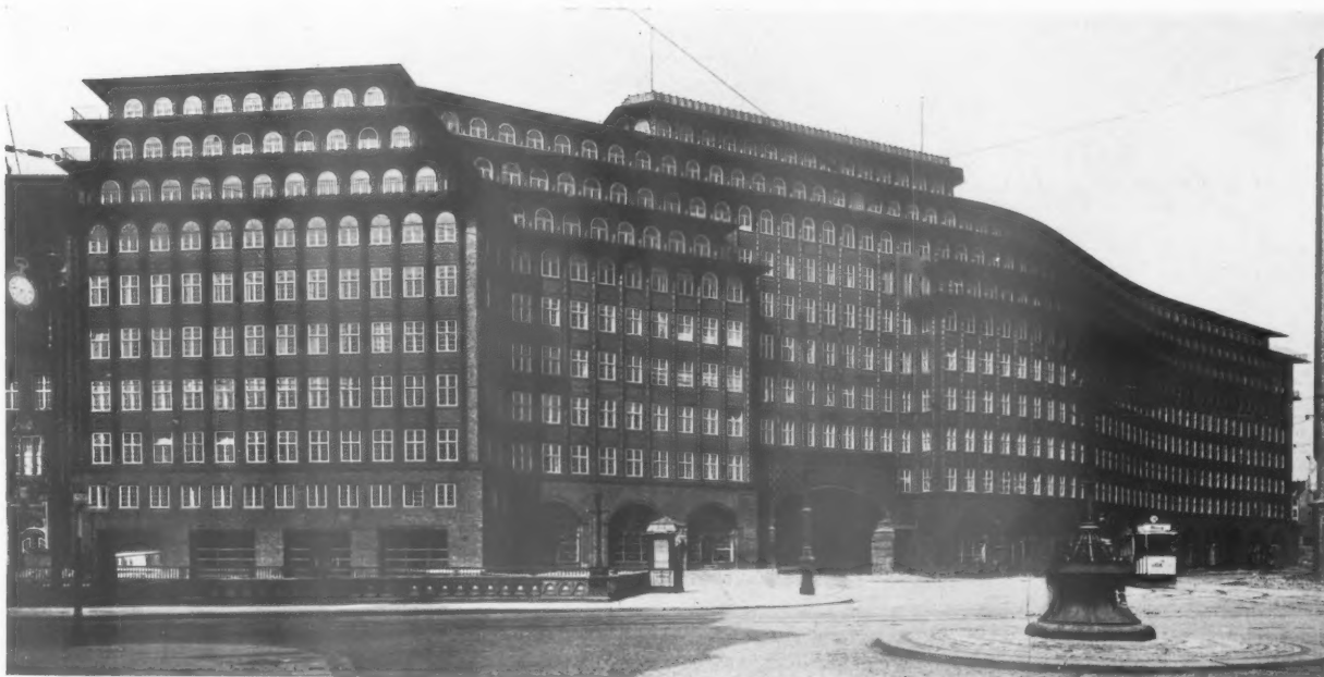
THE FRONT OF THE BUILDING.
