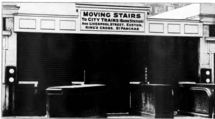
SOUTHERN RAILWAY (SOUTH WESTERN SECTION): Entrance to Escalator, Waterloo Station, fitted with 1 Kinnear Shutter, 9' 6" high by 20' 10" wide.
