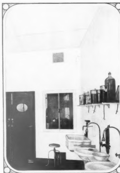
White Vitrolite Wall Lining, in large panels, Ceiling and Shelf to Operating Theatre.
