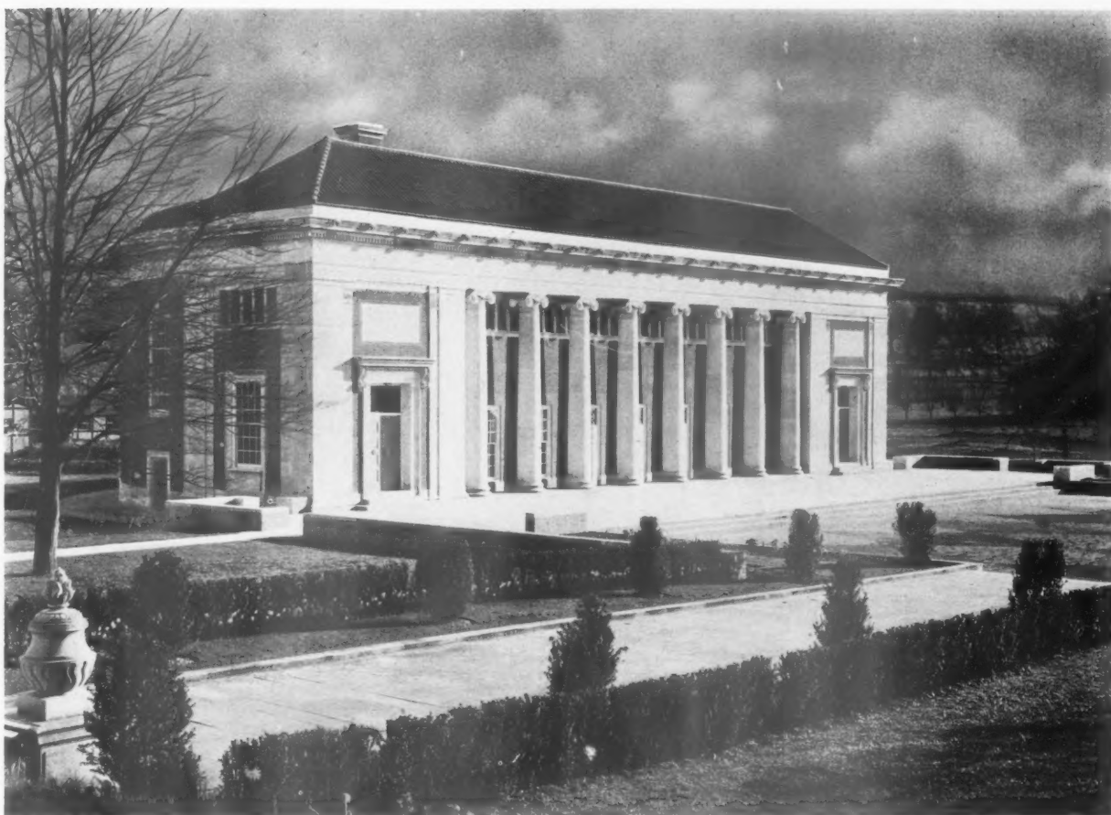
THE HALL, FROM THE NORTH-EAST.
