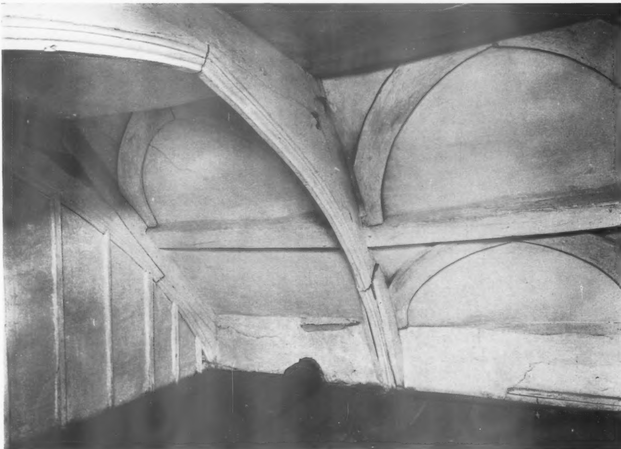
A PORTION OF THE ROOF CONSTRUCTION IN THE BEDROOM, BEFORE RENOVATION. The flat ceilings of the bedrooms were found to be so low that they were removed, and this magnificent roof was discovered above them.
