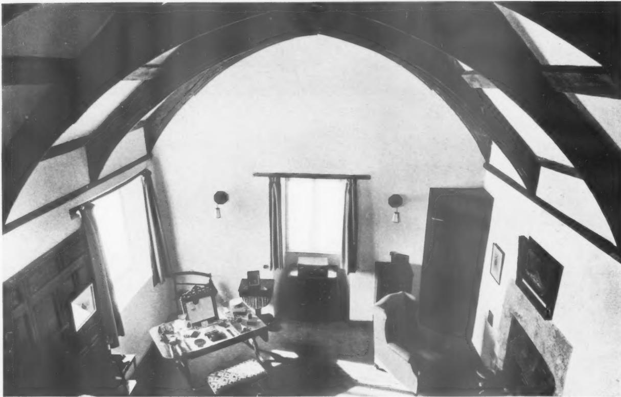
THE BEDROOM OVER THE DRAWING-ROOM. A view taken from an aperture near the ceiling, showing the timbered roof.
