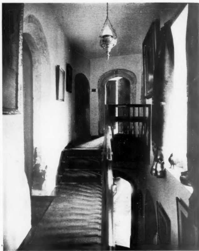
THE STAIRCASE AND FIRST FLOOR.
