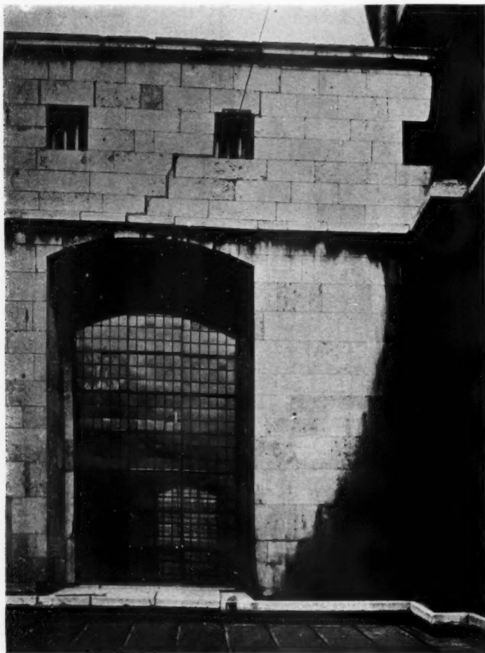
Dislocation of masonry at St. Paul's Cathedral. Right-hand side is dragged down by the weight of the dome. Compare condition of masonry with the statement in the Commission's Final Report.
