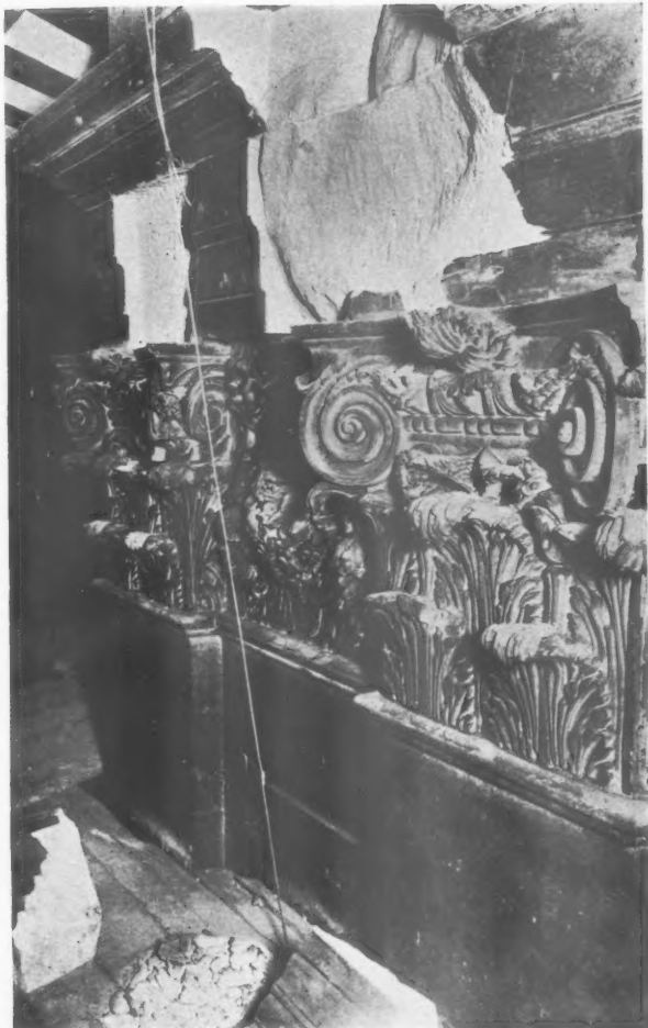
The fractured frieze of one of the piers.
