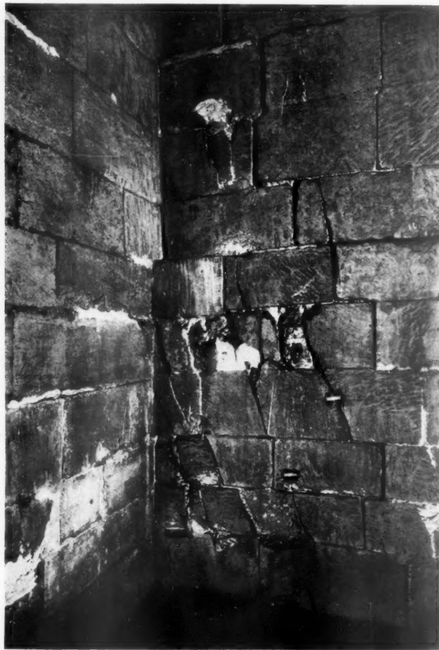
Cracks in the counterforts or buttresses of the drum due to the settlement. These have been filled in. Many years ago it was found that the dome had sunk and was severed from the surrounding mass.
