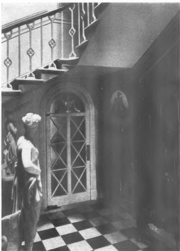
THE STAIR FOOT.
