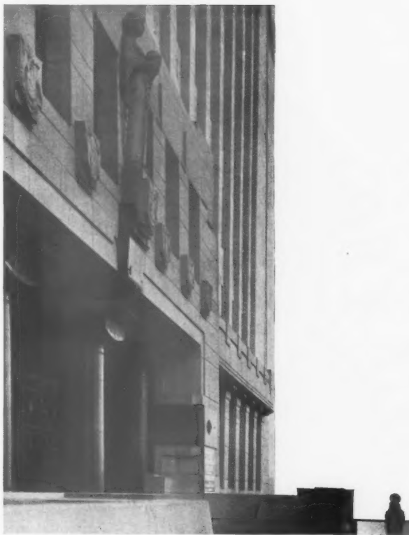
A DETAIL OF THE ENTRANCE.
