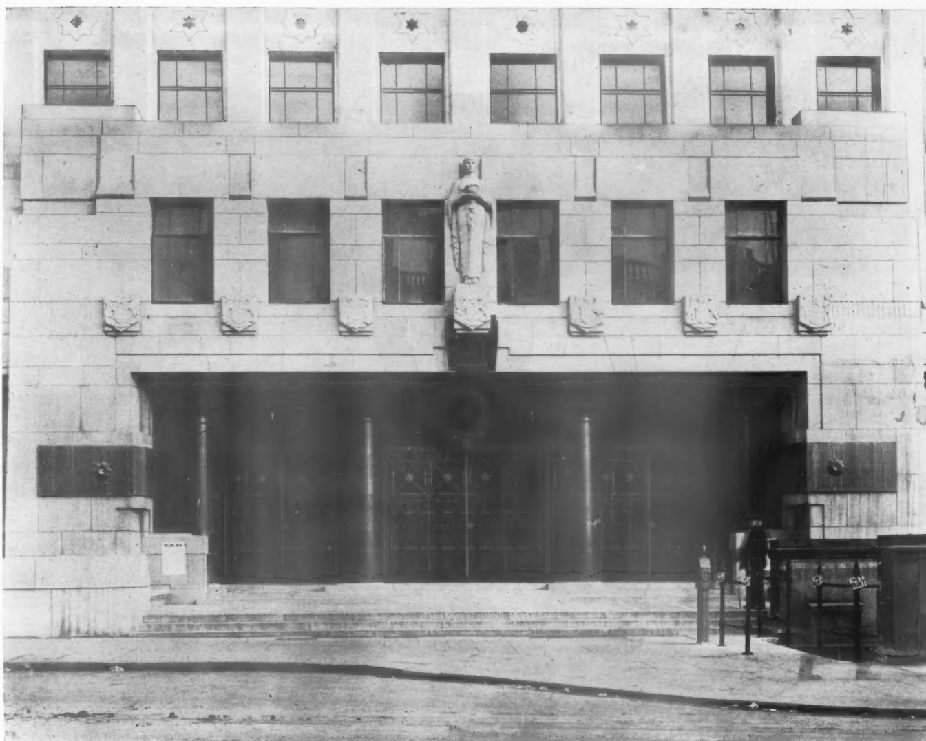
A DETAIL OF THE MAIN ENTRANCE.
