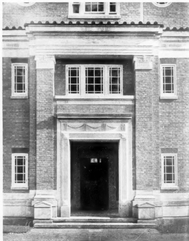
THE ENTRANCE TO THE MAIN BLOCK.
