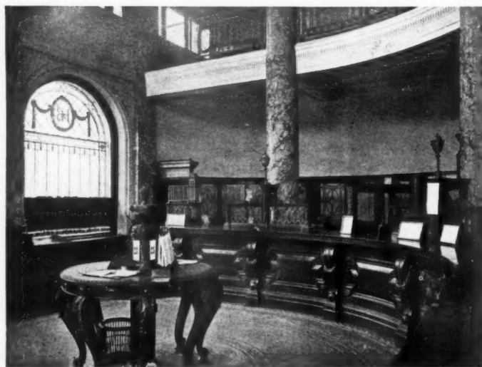
Meers, William H. Bryne & Son, Architects. THE HIBERNIAN BANK, DUBLIN. Scagliola Marble Columns and Pilasters.
