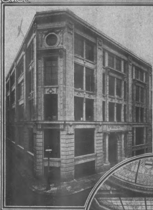
WAREHOUSE—Messrs. Briggs & Co., Ltd. MANCHESTER. Architects: Woodhouse & Dean. Here is a warehouse executed in Vitreous Grey Terra Cotta, from basement to finishing course which shows the possibilities of Terra Cotta.
