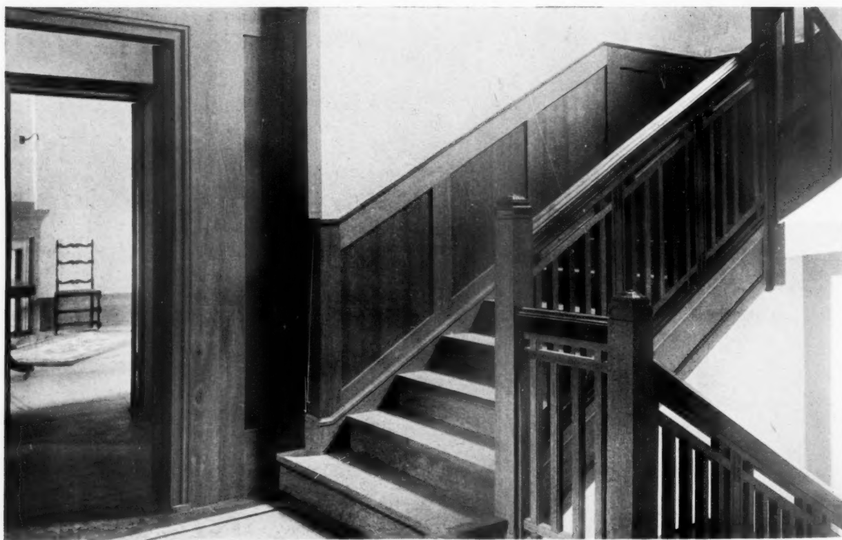
THE STAIRCASE IN THE NEW BUILDING.
