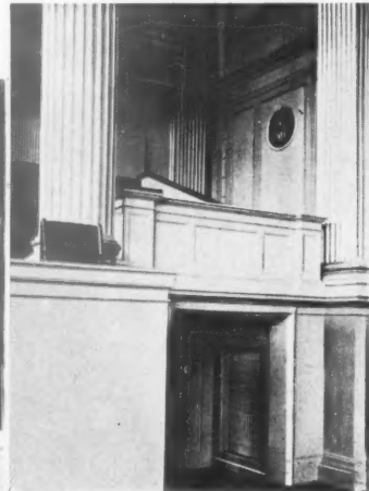
Pre-heated air is supplied through ducts in the cornice while the vitiated air is drawn out through the recessed grille.
