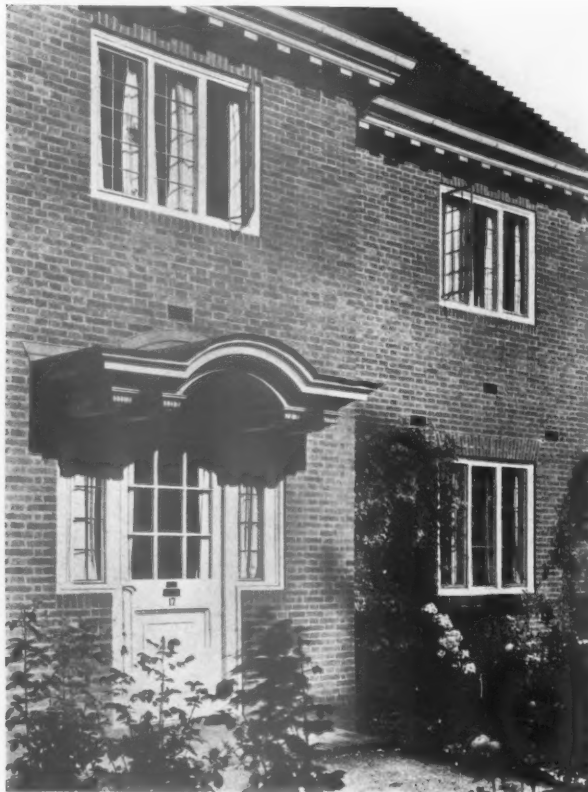
ENTRANCE TO THE NURSE'S HOUSE. The late Ernest Newton, R.A., Architect.
