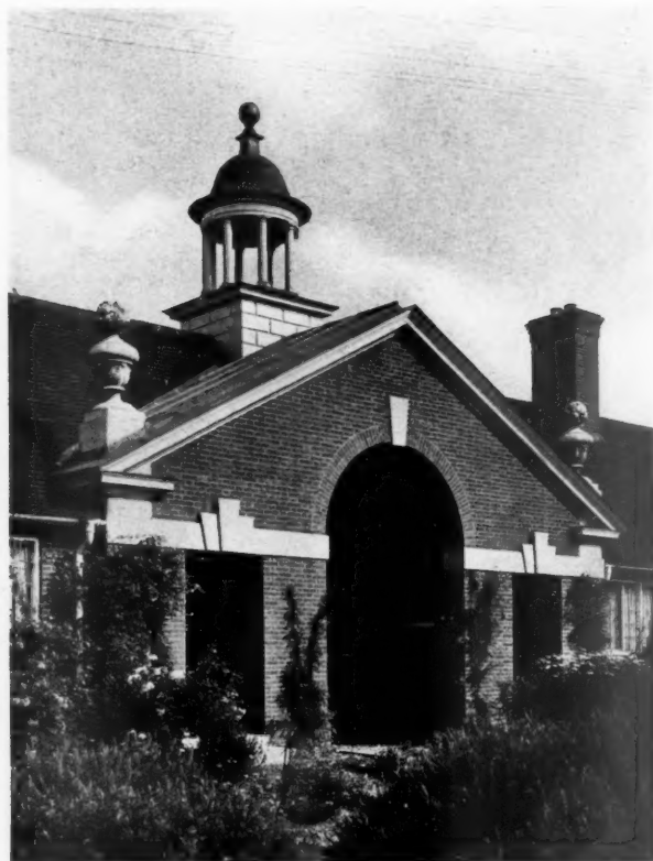
AN ENTRANCE TO A GROUP OF DWELLINGS. Sir Reginald Blomfield, R.A., Architect.
