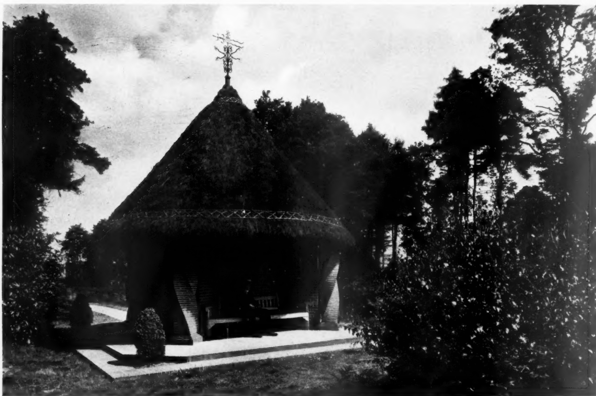
WHITELEY VILLAGE. A SHELTER IN THE GROUNDS. Sheltering the Clerk of Works, Mr. Comport, who has been on duty since the first brick was laid.
