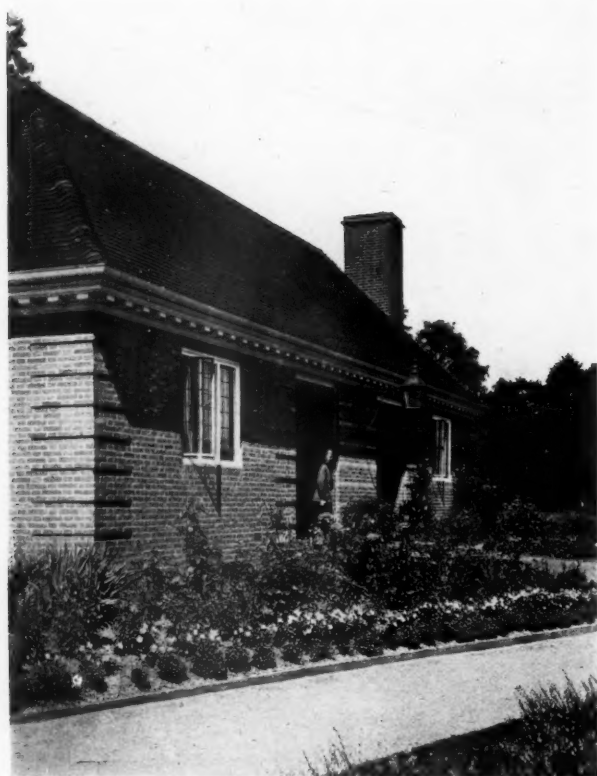
A SINGLE-STORIED DWELLING The late Ernest Newton, R.A., Architect.
