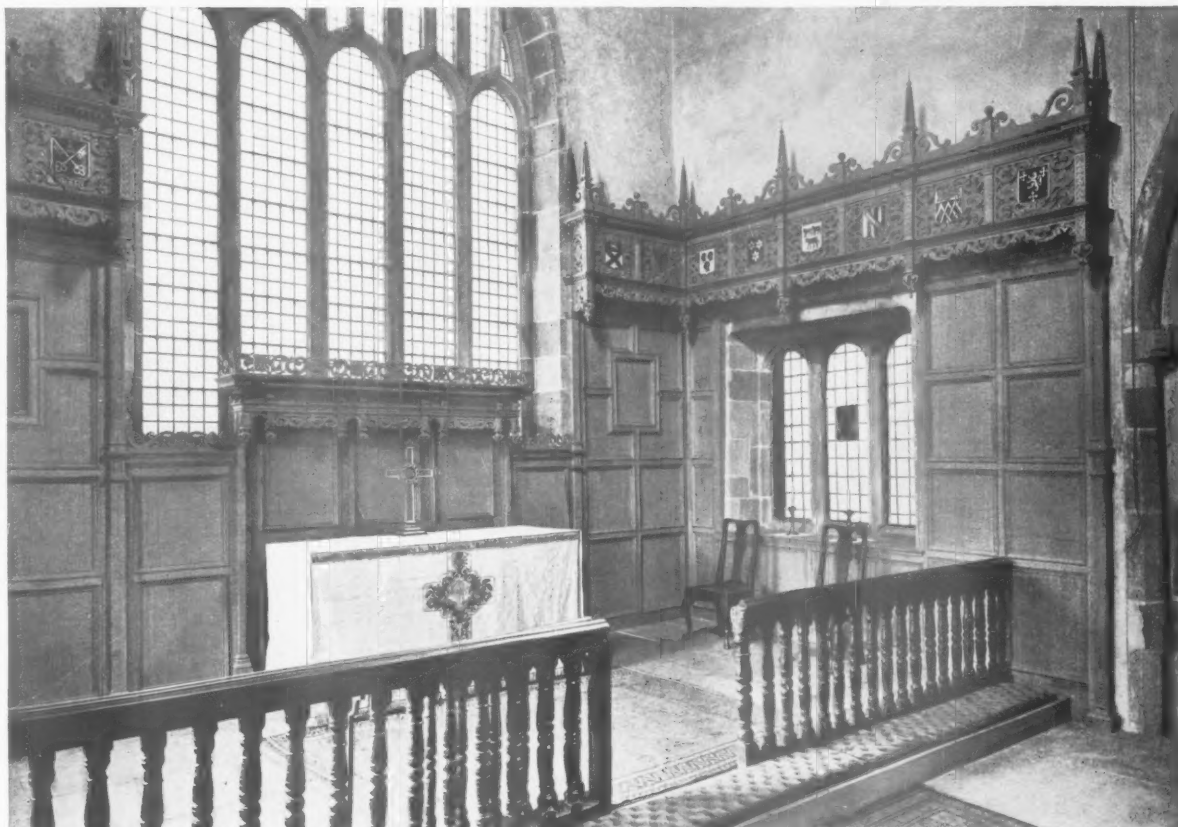
VIEW OF THE SOUTH SIDE.
