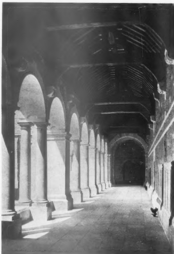
A VIEW DOWN THE NORTH GALLERY.
