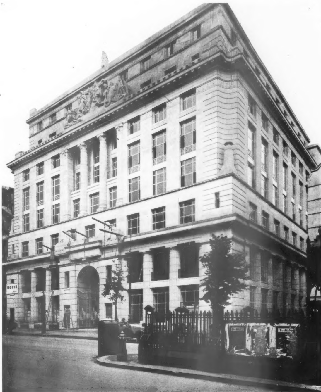
AFRICA HOUSE, KINGSWAY.
