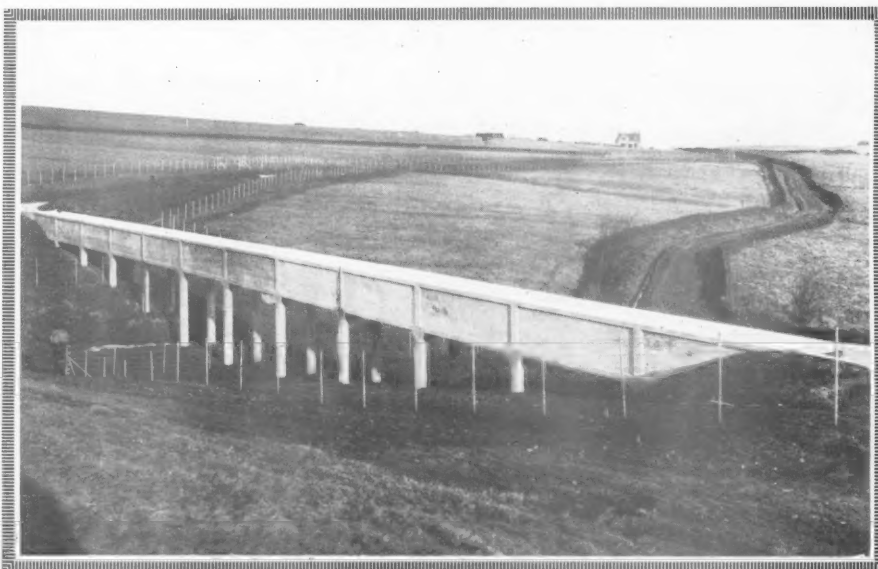
Aqueduct, Loch Coulter Water Works, Denny, Stirlingshire, for Stirlingshire & Falkirk Water Works Engineers: Messrs. Warren & Stuart Reinforced entirely on B.R.C. system
