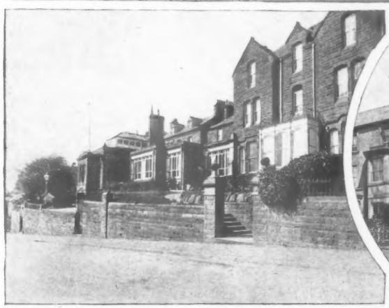
Oldham House Hydro, Macclesfield
