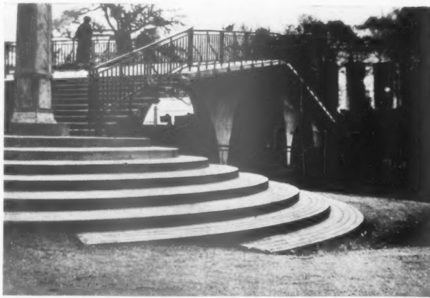
12. A CONCRETE BRIDGE ACROSS THE LAKE.
