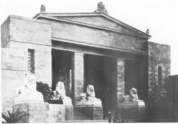
2. THE GOVERNMENT BUILDING. Built of breeze blocks finished in cement mortar.
