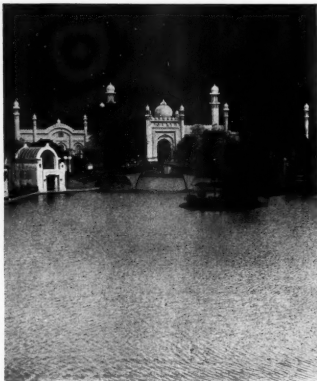
INDIA, FROM A BRIDGE.
