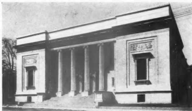
4. THE ART ASSOCIATION BUILDING, MONTREAL.
