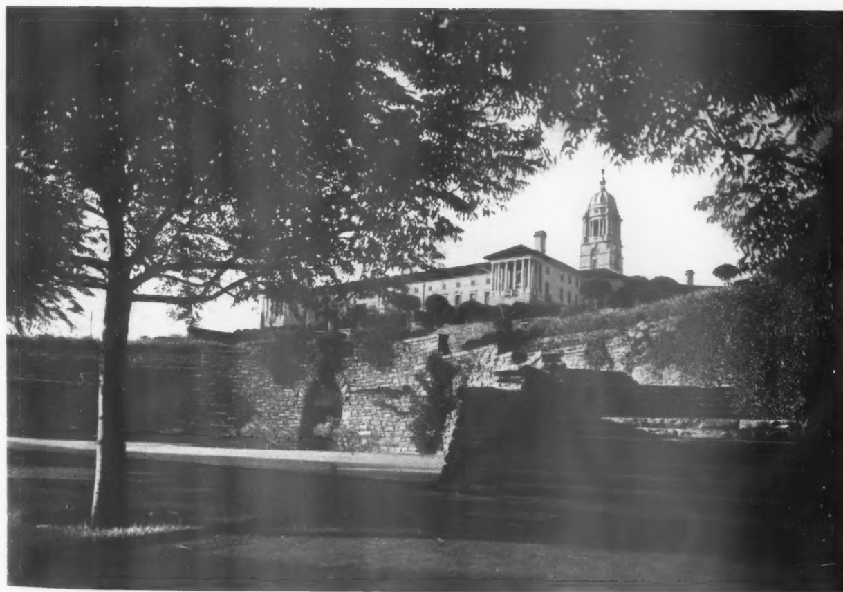
UNION BUILDINGS, PRETORIA. Designed by Herbert Baker.
