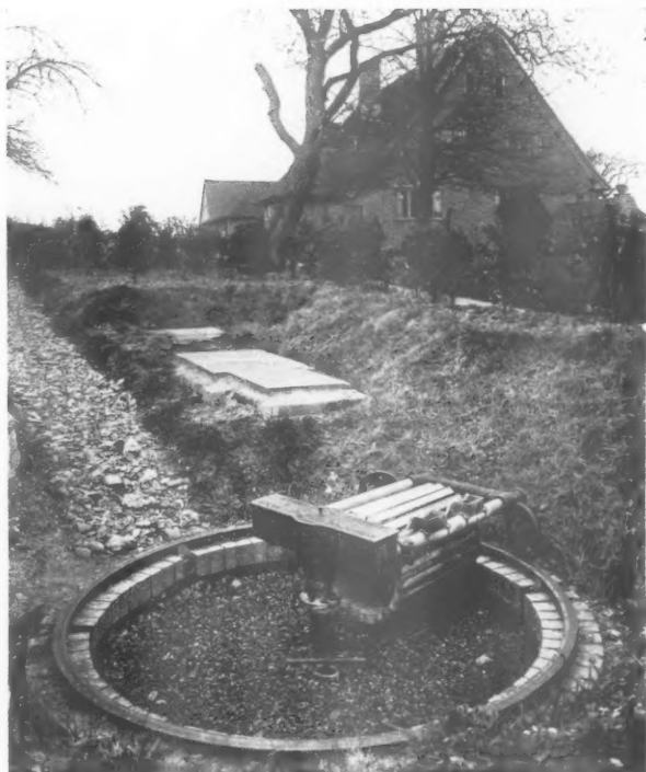
Small Sewage - disposal Plant installed for Henry J. Hare, Esq., Past-President, R.I.B.A.
