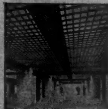
Admiralty Stores, S.W. Pavement Lights in Light Well.
