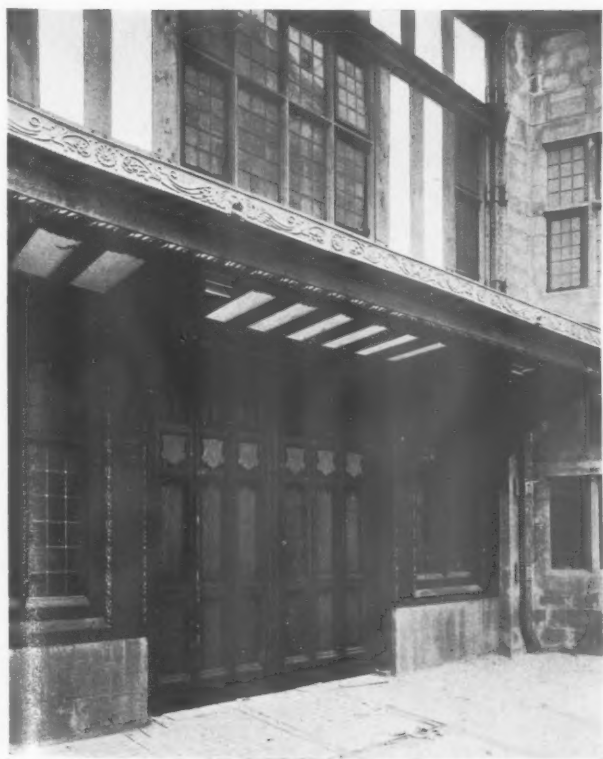
THE FRONT ENTRANCE.
