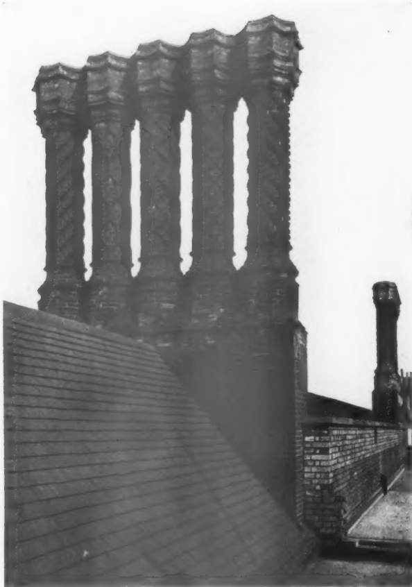
CHIMNEY STACKS ON TUDOR HOUSE.
