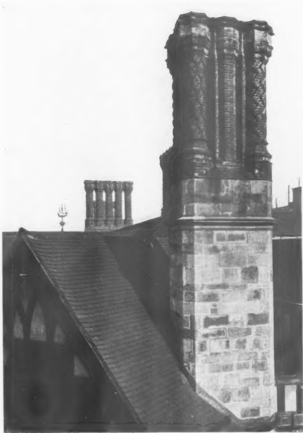
CHIMNEY STACKS ON TUDOR HOUSE.
