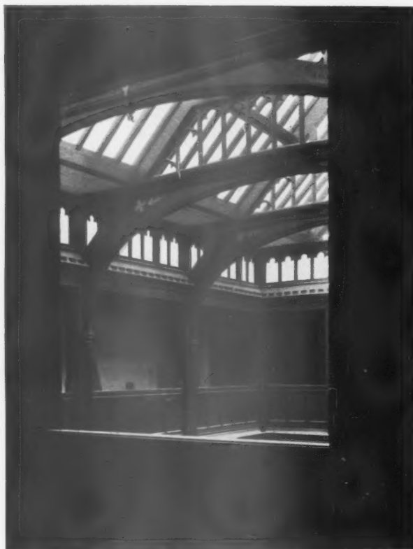
THE SKYLIGHT TO THE WEST WELL.
