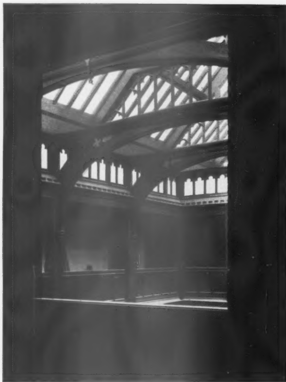
THE SKYLIGHT TO THE WEST WELL.
