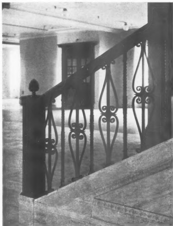
A DETAIL OF THE STAIRCASE BALUSTRADE.
