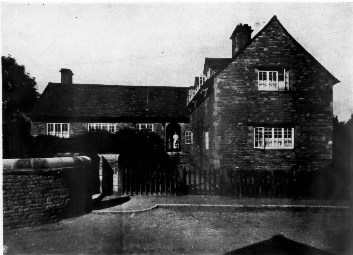
THE HALL LAUNDRY.
