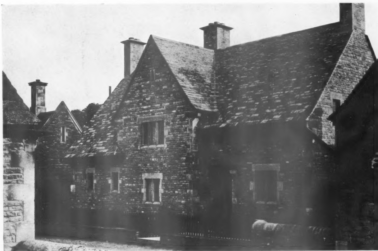
THE CLERK OF WORKS' HOUSE.
