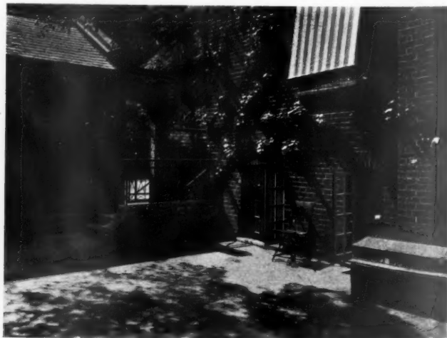
THE ENTRANCE GATE FROM THE COURTYARD.
