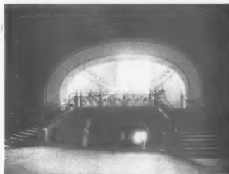
WESLEYAN CENTRAL HALL, MESSRS. LANCHESTER & RICKARDS, FF.R.I.B.A., Architects
