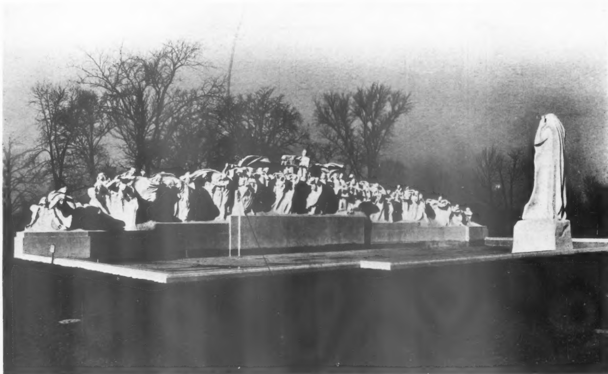
A GENERAL VIEW OF THE FOUNTAIN OF TIME.
