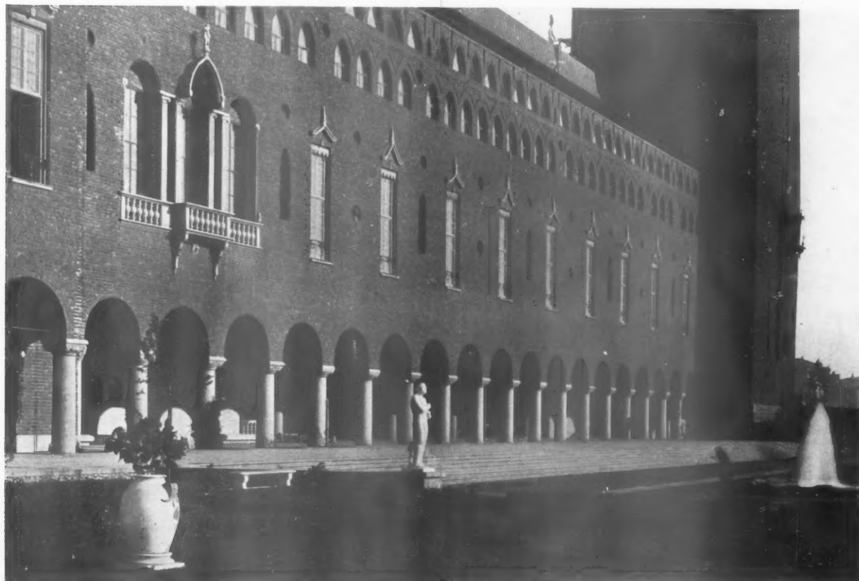
THE SOUTH FRONT FACING THE LAKE.
