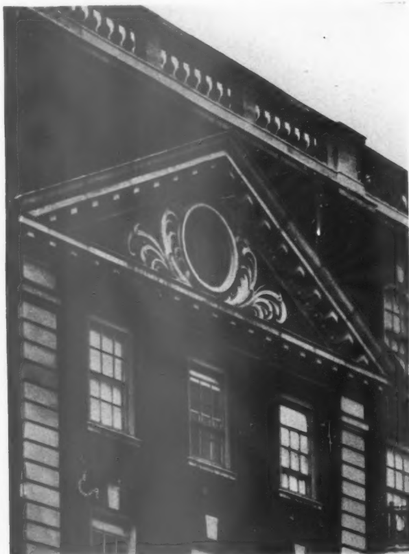
A DETAIL OF THE PEDIMENT.
