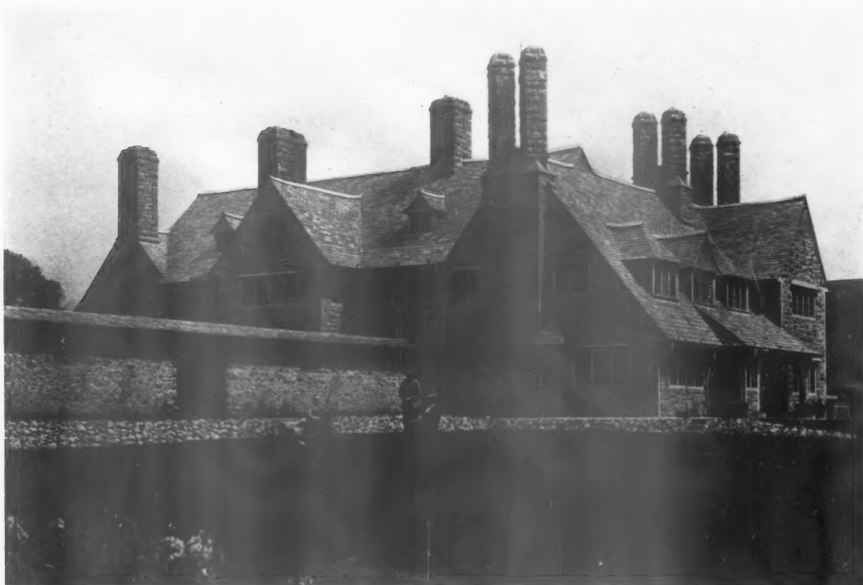
WINTERFIELD FROM THE SOUTH-WEST.
