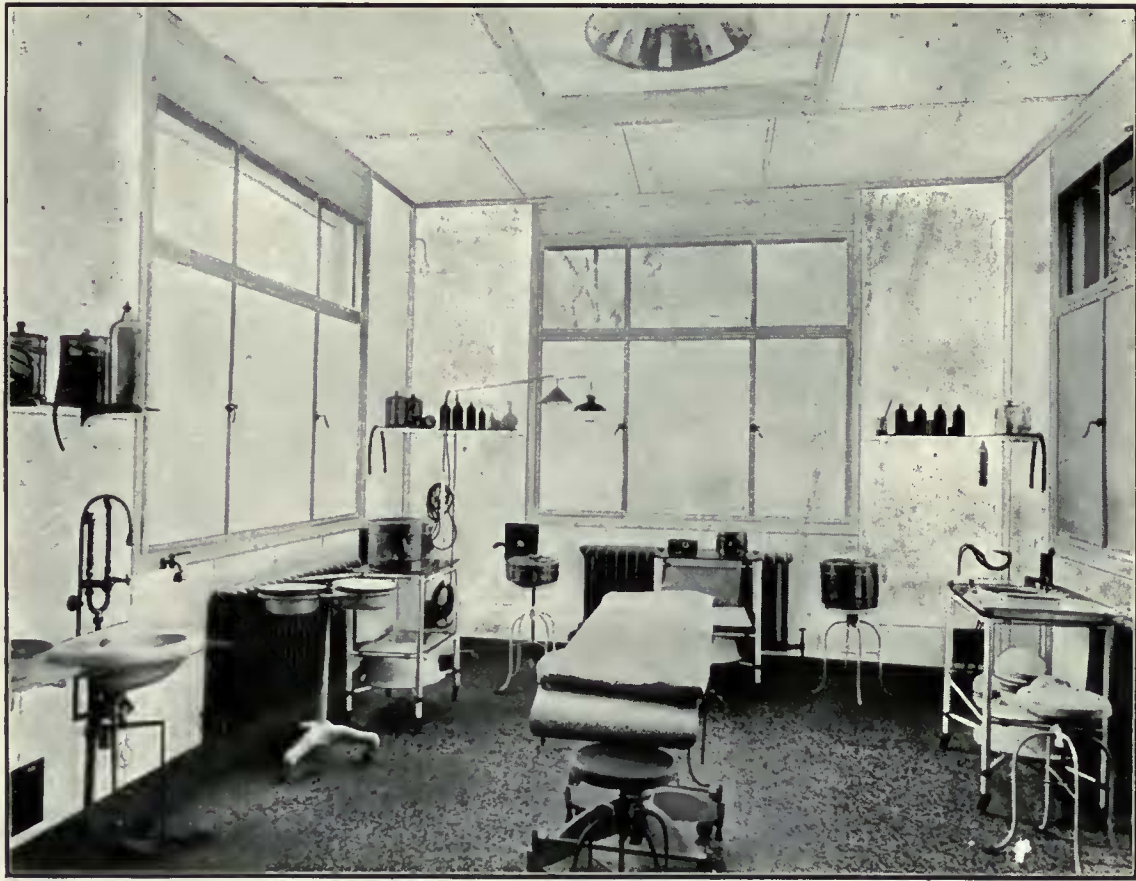
Operating Theatre, St. John's Hospital, Lewisham, showing complete Vitrolite installation comprising walls, ceiling, shelving, instrument cupboards, etc.
