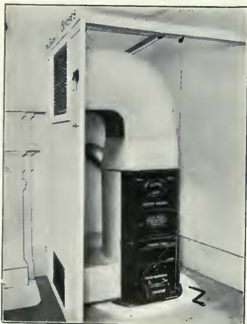
A typical installation of the small British Wonder Heater taken in our showroom in order to show positions of warm-air outlet at top, cold-air inlet at foot, and the simple arrangement in the hall or room to open or close dampers to regulate the temperature without trouble.
