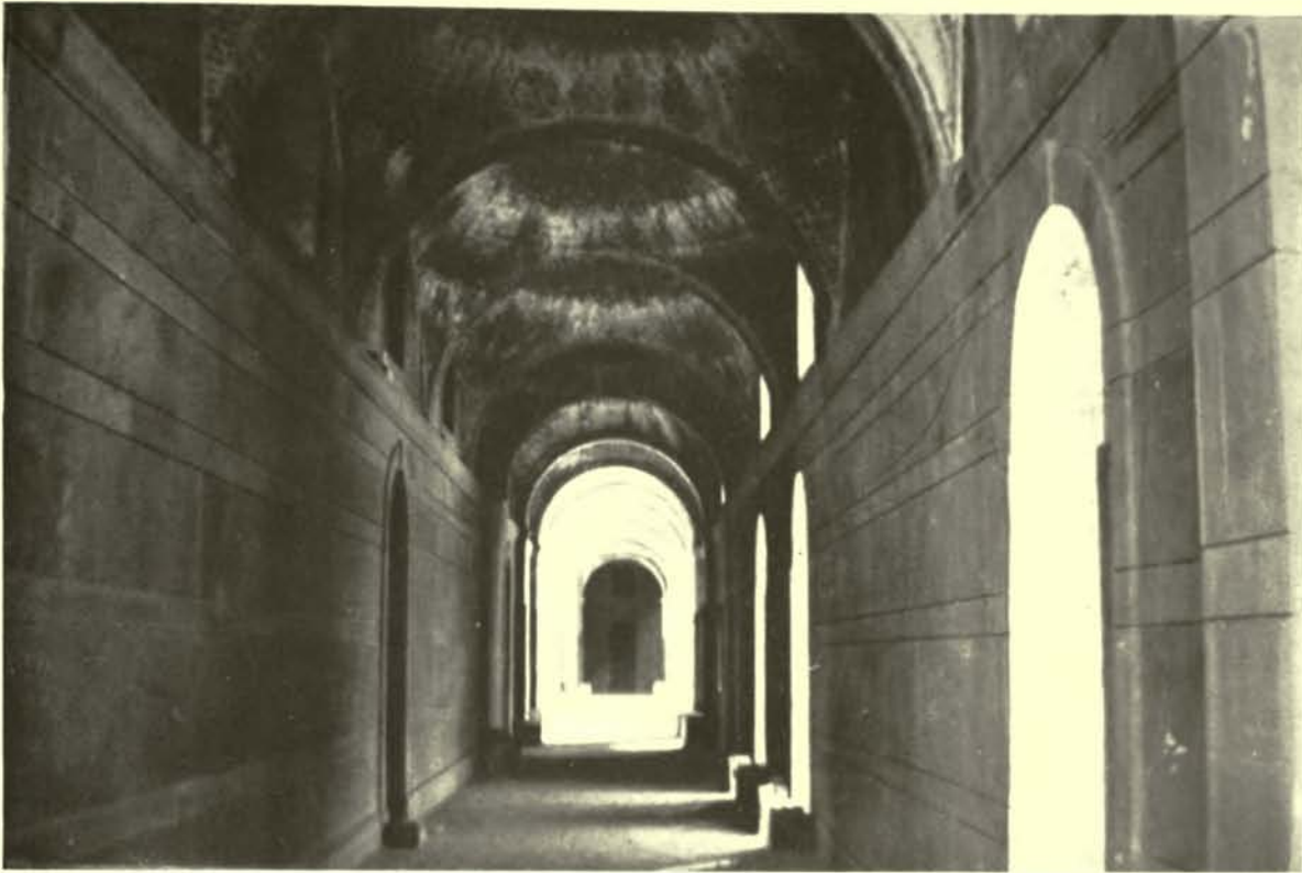
9.—TYPICAL CORRIDOR WITH DOMICAL VAULTING.
