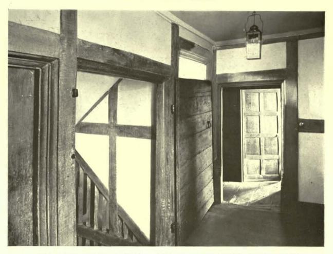
THE FIRST-FLOOR LANDING, AND SOLID MOULDED DOOR-FRAMES.
