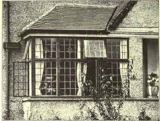
Hayward's Patent "Putty Grooved" Steel Casements and "Prior" Lead Glazing.
