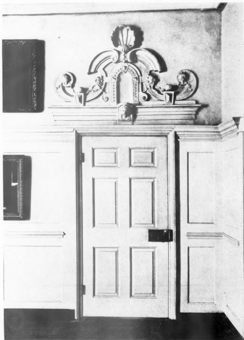
DOORHEAD IN THE KING'S DINING-ROOM, KEW "PALACE."
