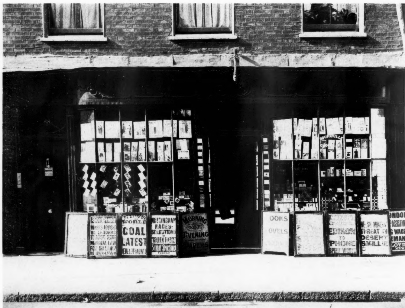
DOUBLE-FRONTED EIGHTEENTH-CENTURY SHOP-FRONT, No. 88 DEAN STREET, W.
