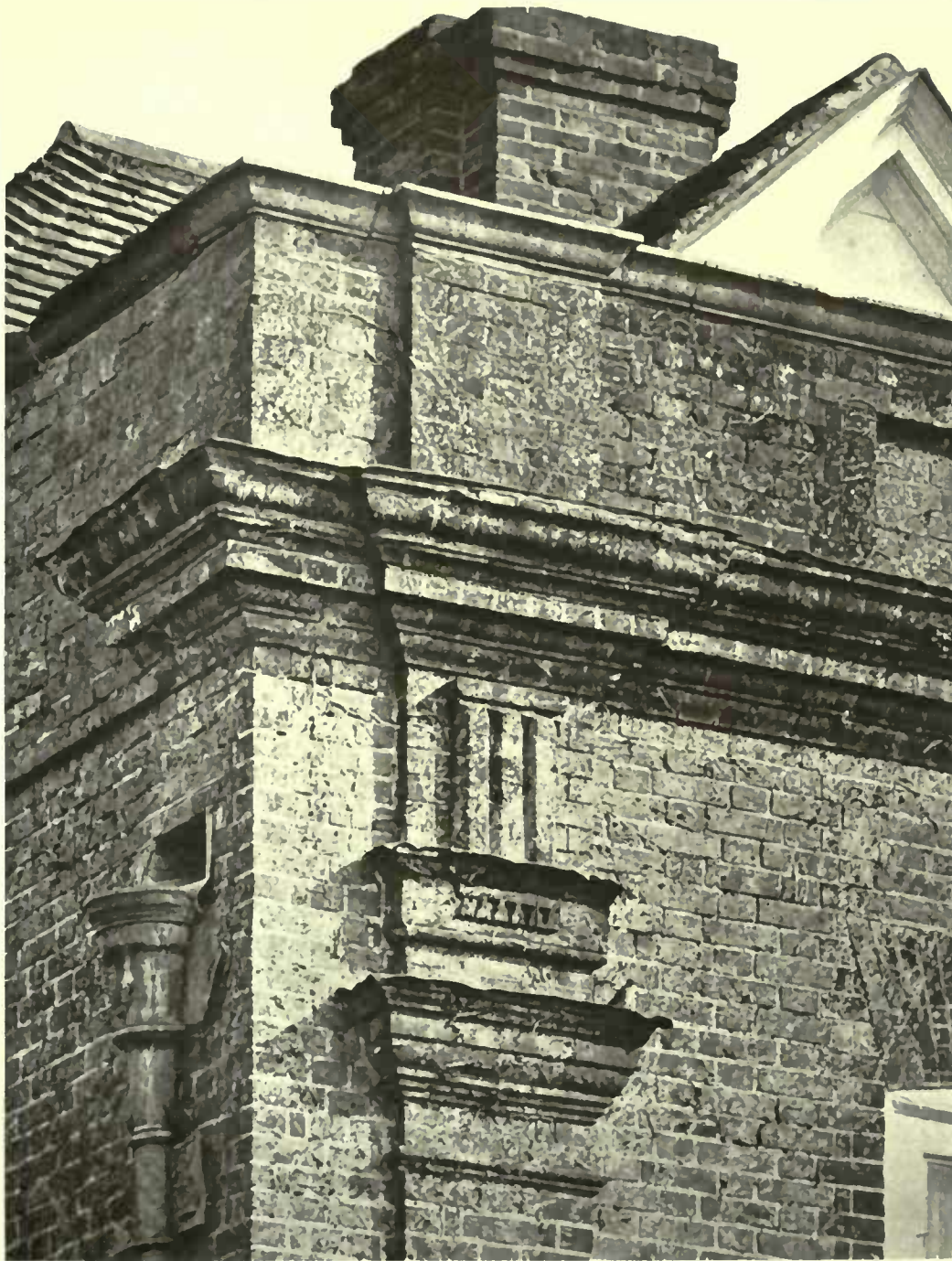
DETAIL OF MOULDED BRICKWORK ON NORTH FRONT.
