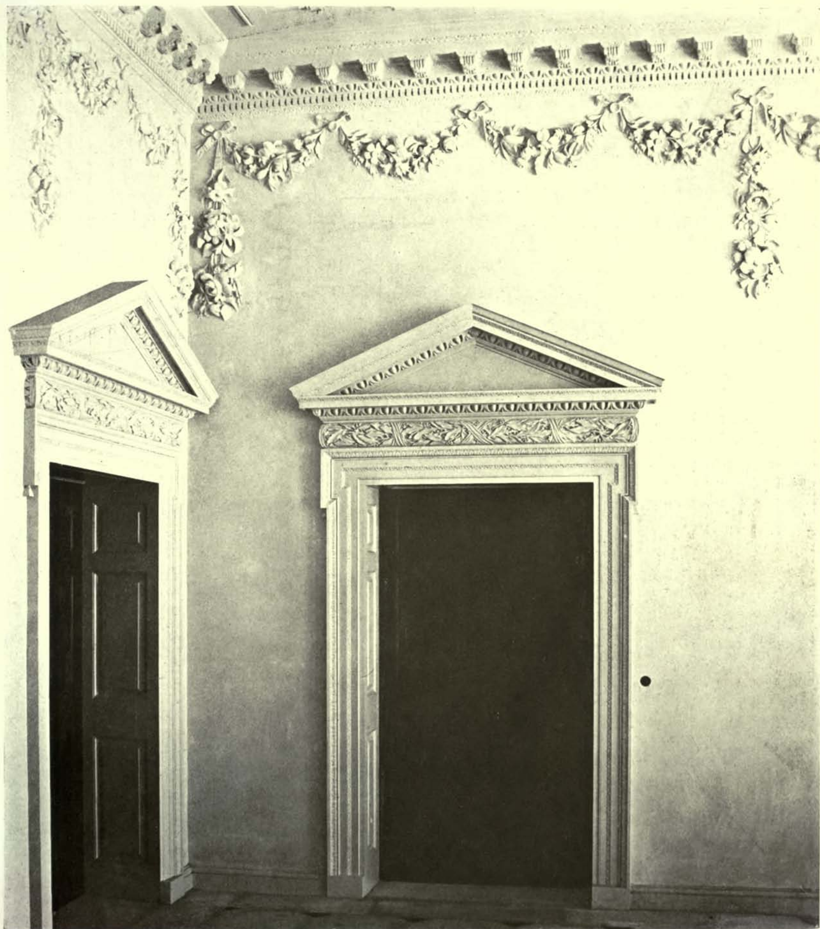
The doors are of solid mahogany, with surrounds of deal, and cast enrichments ; plaster cornice and wall decorations.
